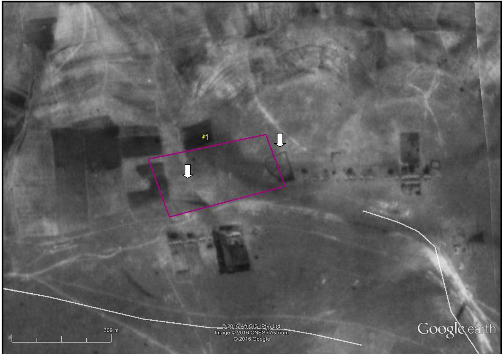
FIG. 8: AERIAL PHOTOGRAPH OF BORROW PIT 1 IN 1954
