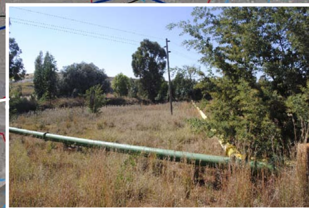
014: North-easterly view of pipeline route
