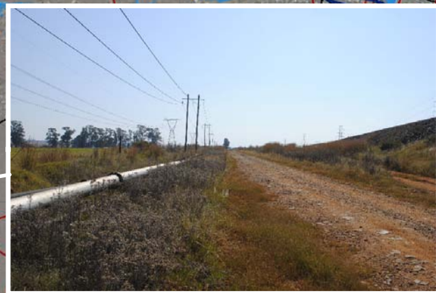
004: Northern view of pipeline route
