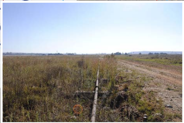
008: Northern view of pipeline route
