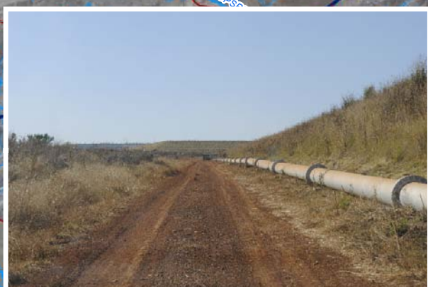
046: Northern view of pipeline route
