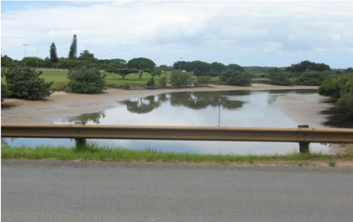
Plate 2 Medway Road Bridge over the Ngodweni River
