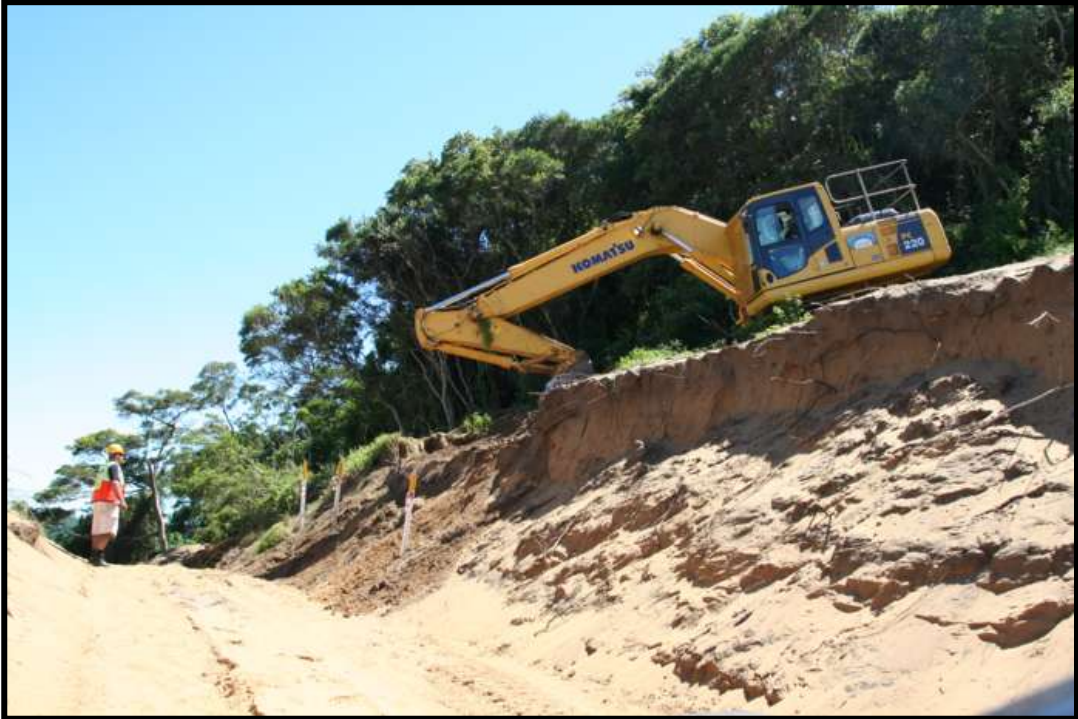
Fig. 20: Excavator Removing Topsoil at MPE139
