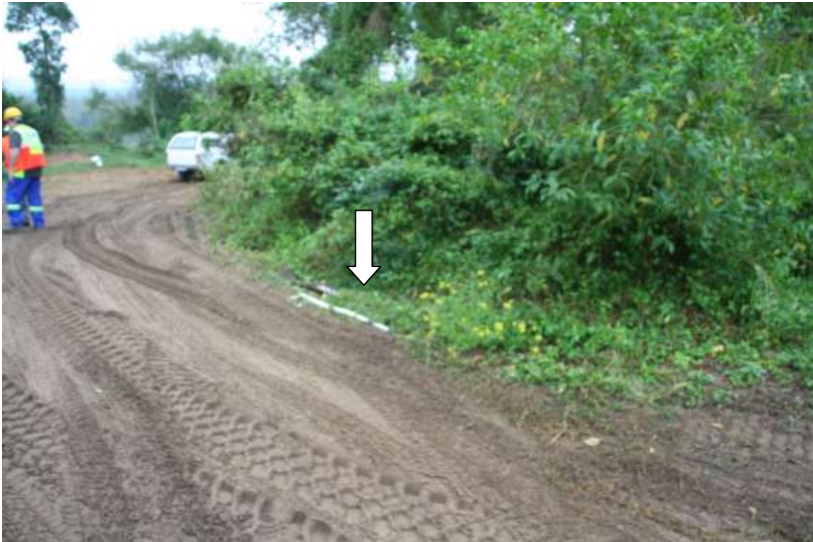
FIG. 4: REMOVED GREEN WOODEN POLE
