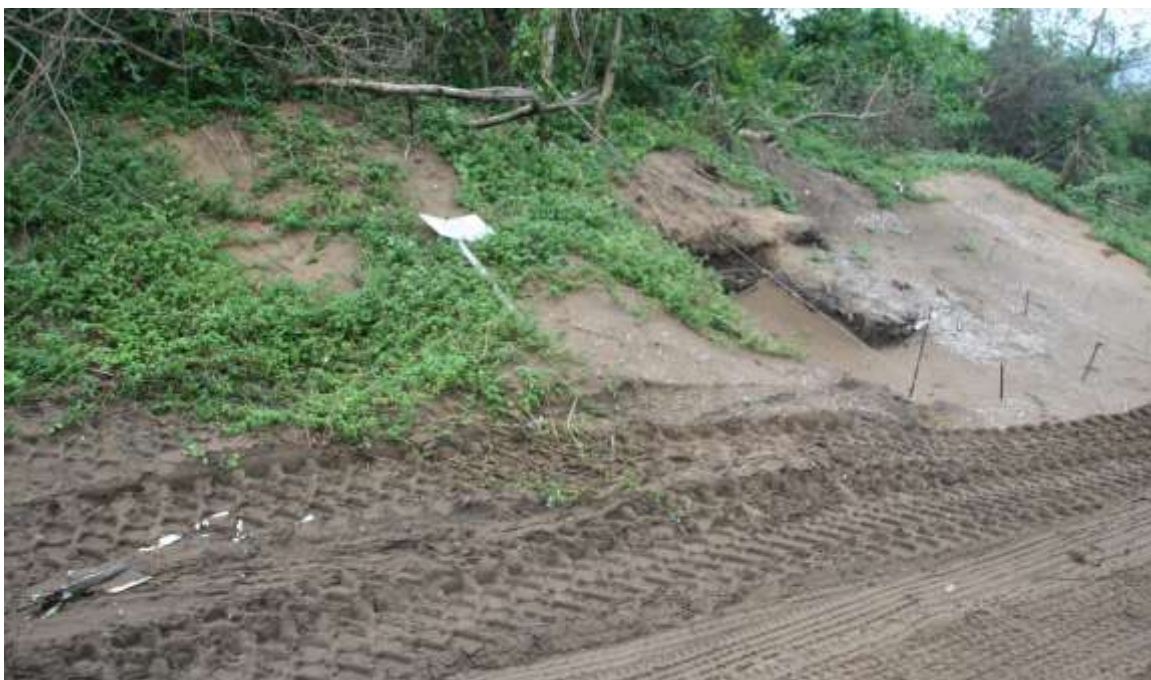
FIG. 5: CRUSHED WOODEN POLE, METAL SIGNAGE REMOVED TO ONE SIDE, TRACKS NEXT TO EXCAVATIONS
