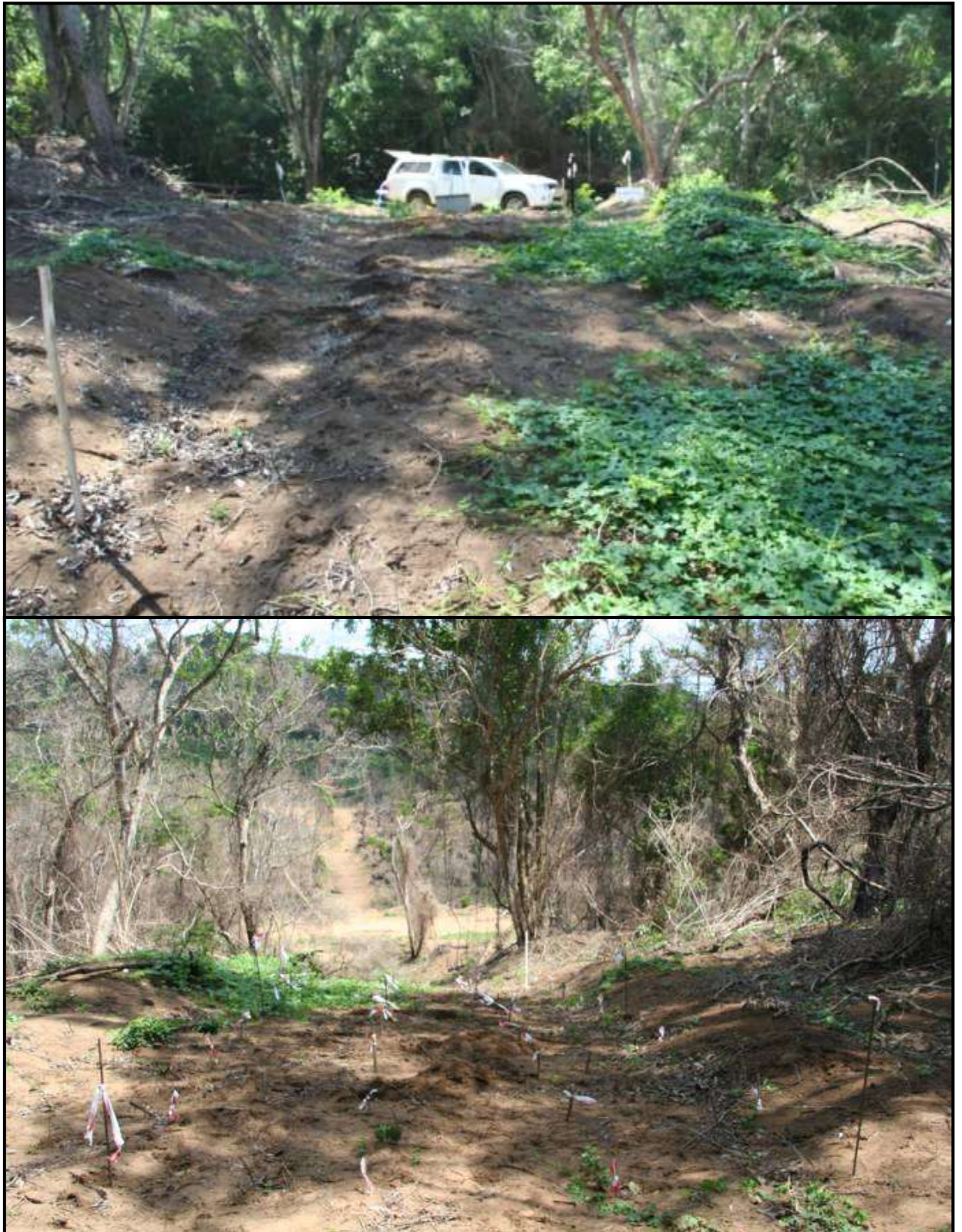
Fig. 21: General View Of The November 2014 Excavation Area
