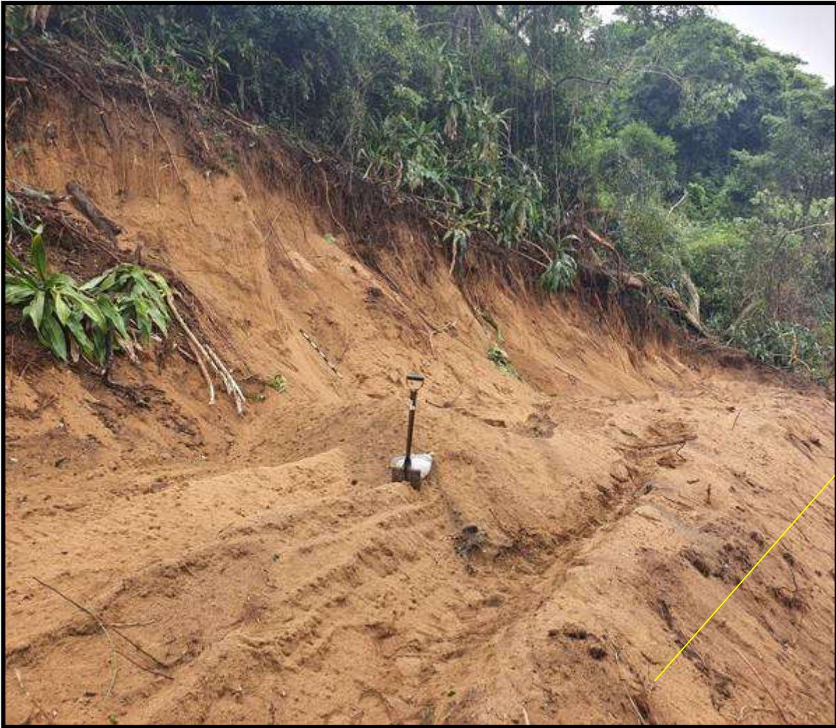
FIG. 44: TOPSOIL REMOVAL 1
