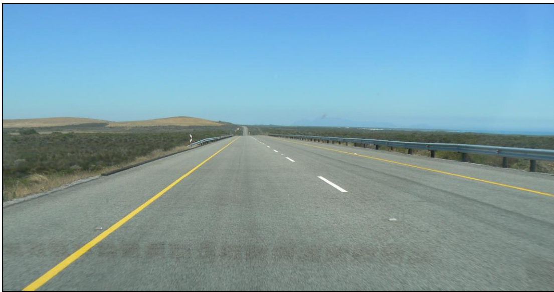
FIGURE 37: R 27 between the R 315 intersection and Blaauwberg
