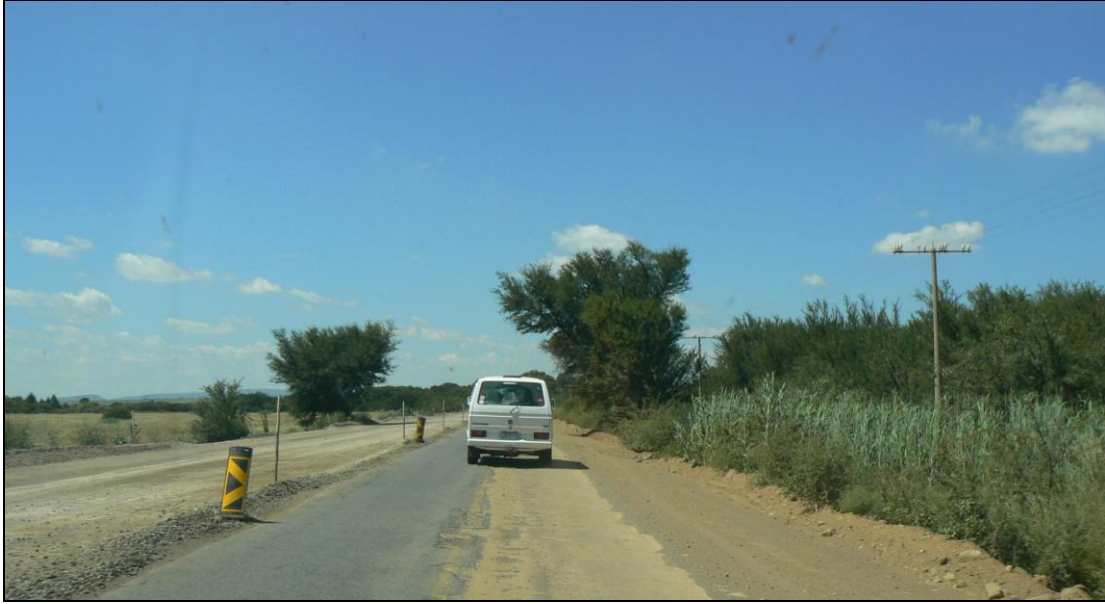
FIGURE 12: The N 6 between Reddersburg and Smithfield is being widened and rebuilt
