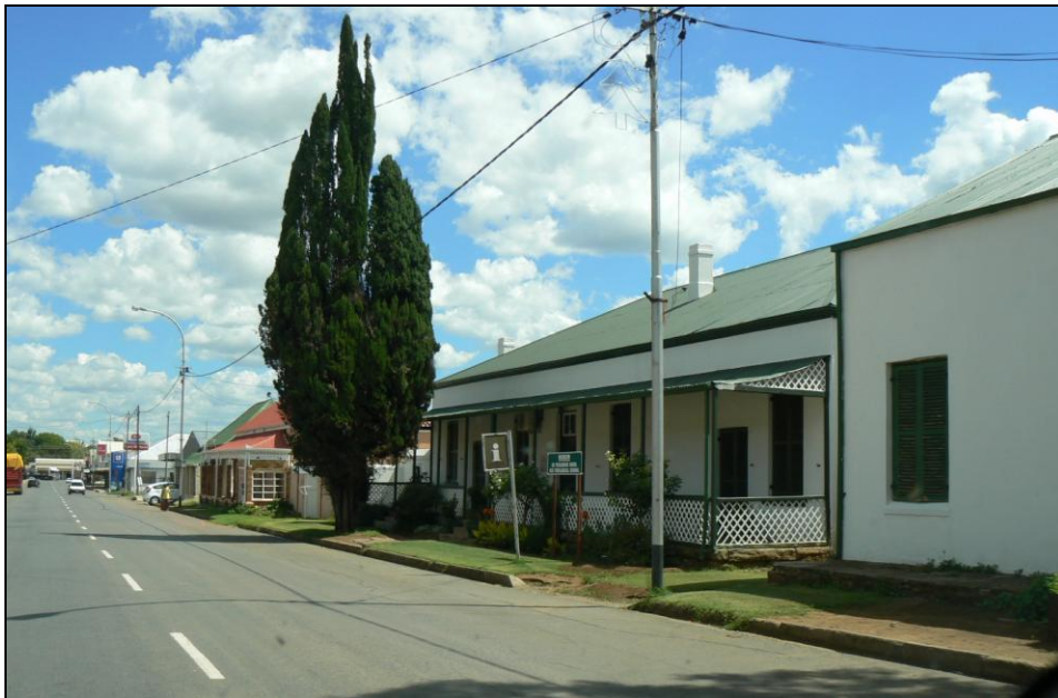
FIGURE 43: Various historic buildings front on Piet Retief and other streets in Burgersdorp
