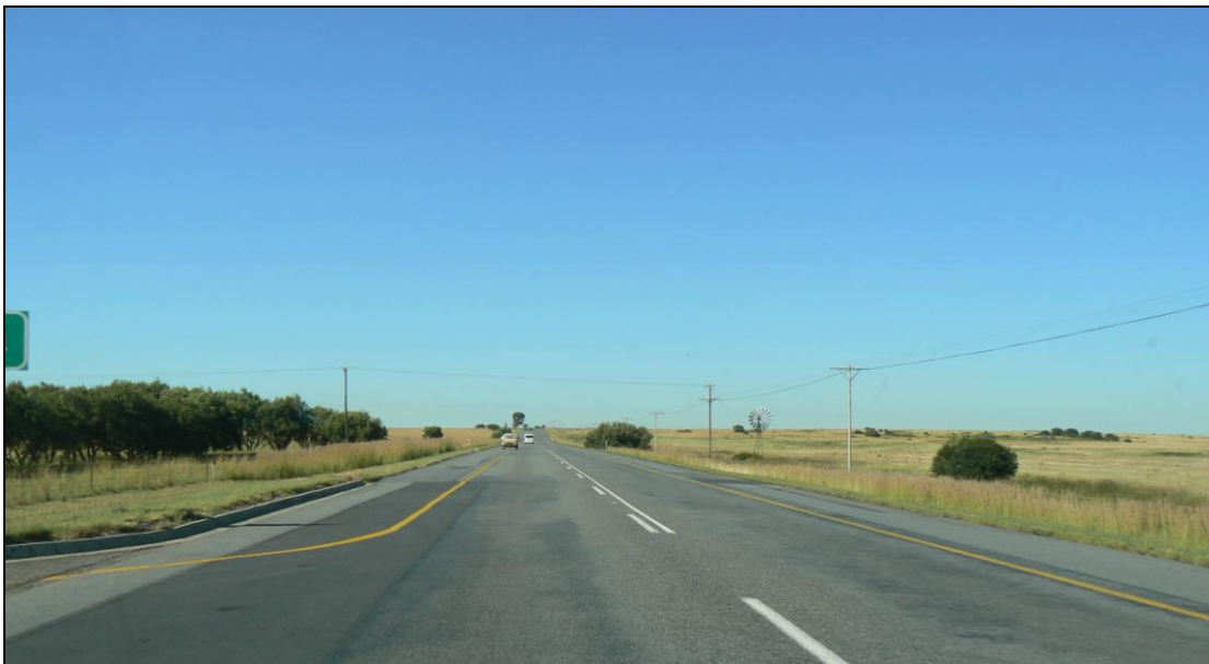
FIGURE 5: Kroonstad-Ventersburg section of the N 1
