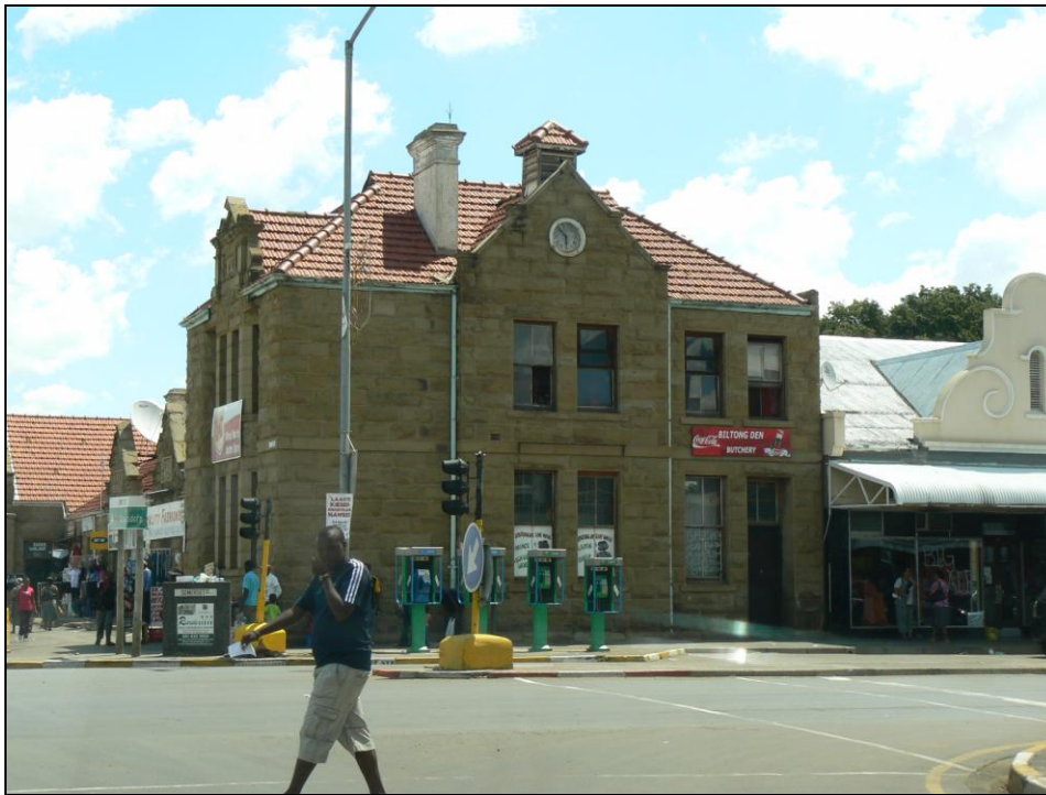
FIGURE 42: The former magistrate's and post office (1896) on the corner of Grey and Smith streets is one of Aliwal North's most important historical buildings
