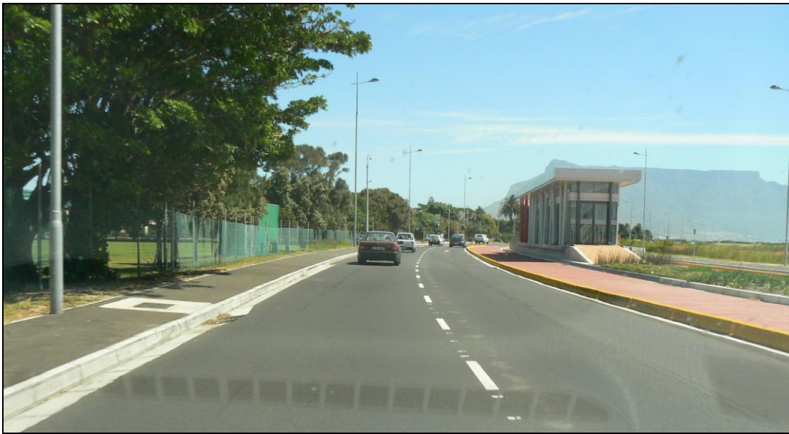
FIGURE 36: Table View section of the R 27 with one of the completed BRT stations
