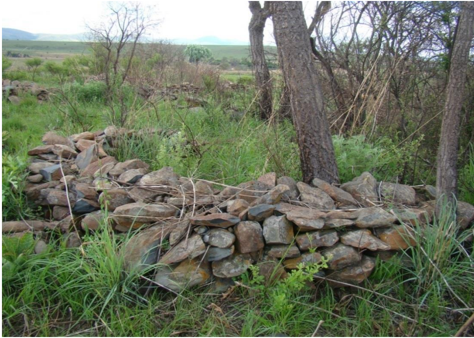
Photo 65: This specific circular wall is still in a very good condition.
