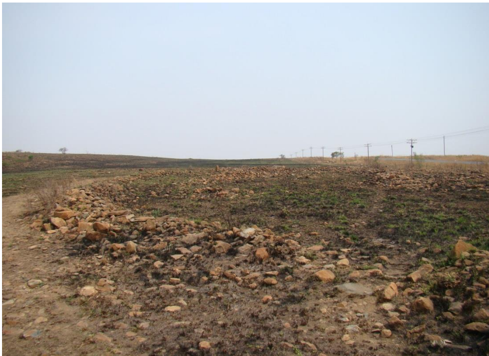
Photo 58: RDR1 G has been impacted upon by the tarred road (R36) which cuts through this unit. The walls are not generally in good condition.
