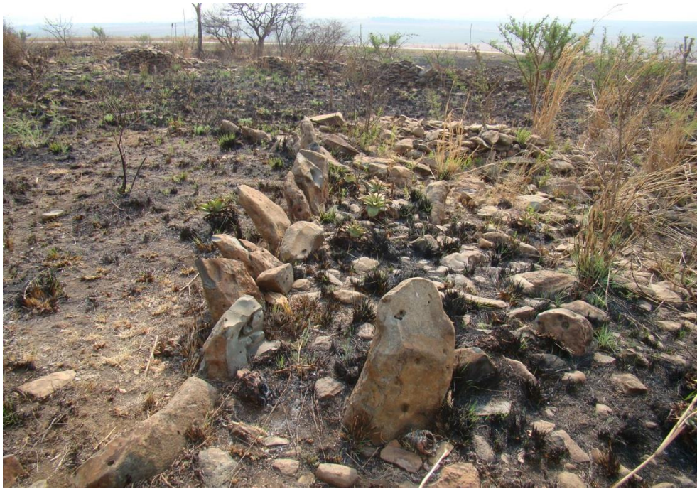
Photo 69: Large foundation stones are also distinct in this section.
