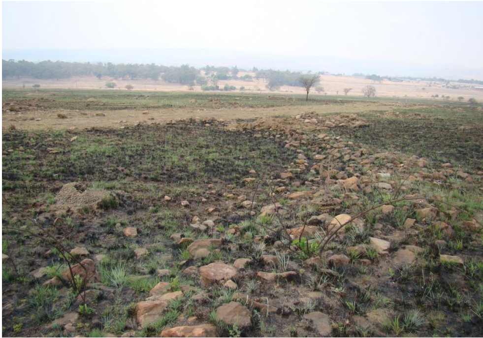
Photo 47: The condition of the walls is visible in this picture.
