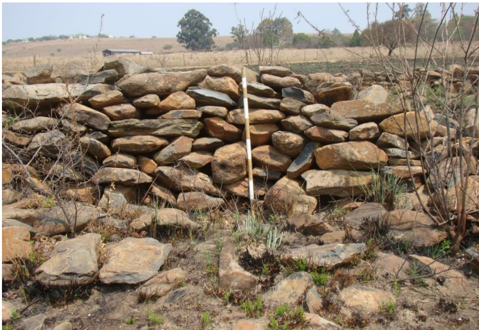
Photo 24: Section of the wall that is 800mm high.
