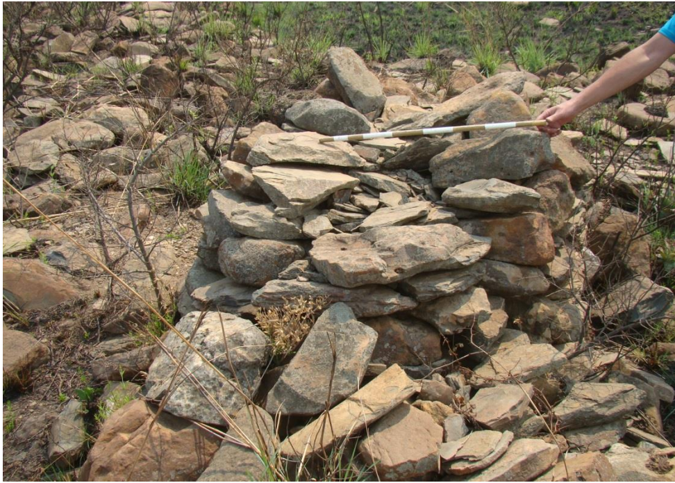
Photo 31: The same section of this wall is over 1000mm wide.
