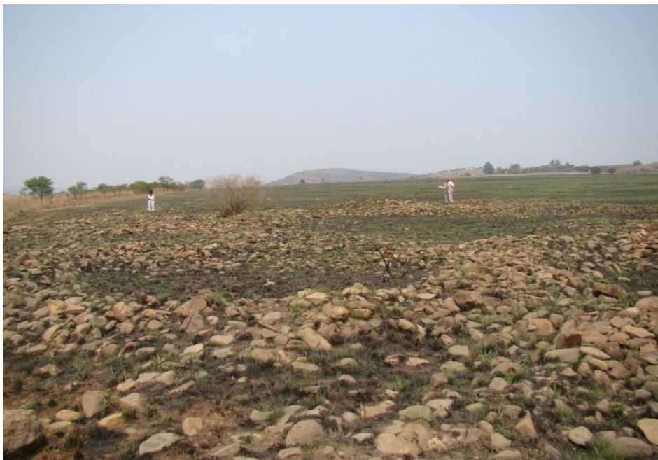
Photo 41: Unit RDR2C unit is further north of RDR2A, B & C. It is well defined. Highest section: 300mm, but deteriorating fast.
