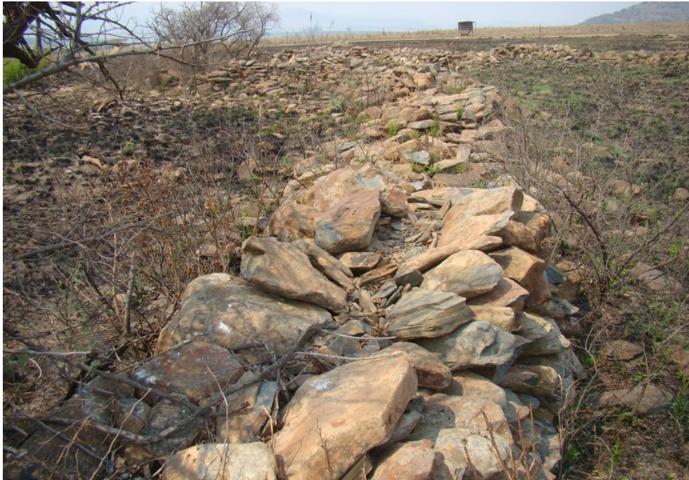
Photo 25: The typical building method of the LIA stone walls is visible with the larger stones on the outside filled in with smaller stones.
