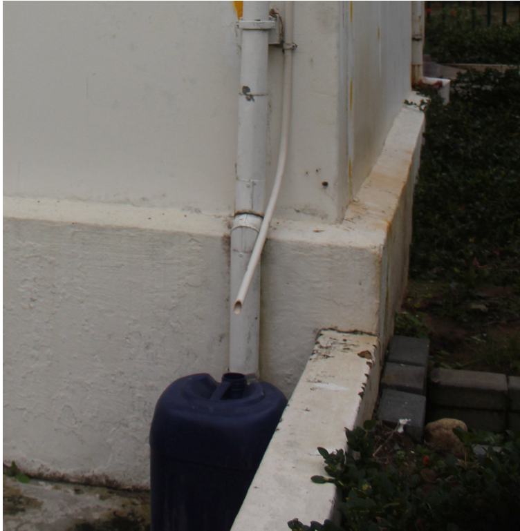
Fig. 7: All surrounding moisture sources to be removed
