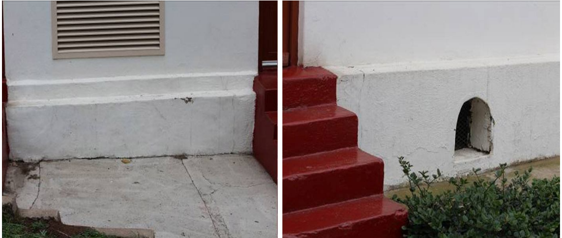
Fig.11: Substantial concrete plinth Fig. 12:Underside vent on south side
