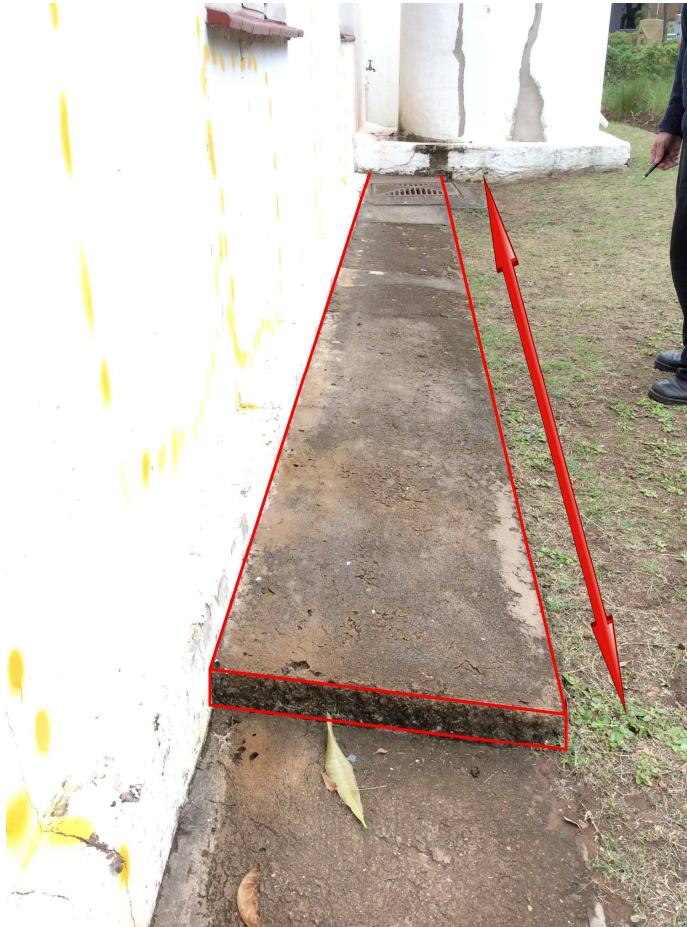
Fig. 14: Section to be lowered
