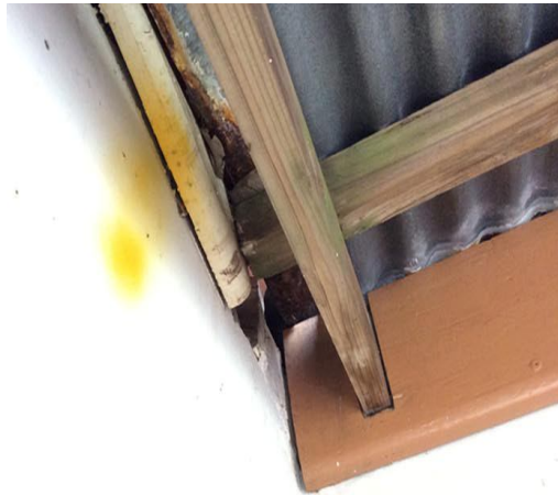
Fig. 3: View from verandah
