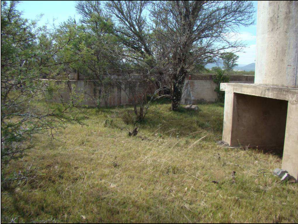
Fig.16 Reservoir tanks and dams at Point R.
