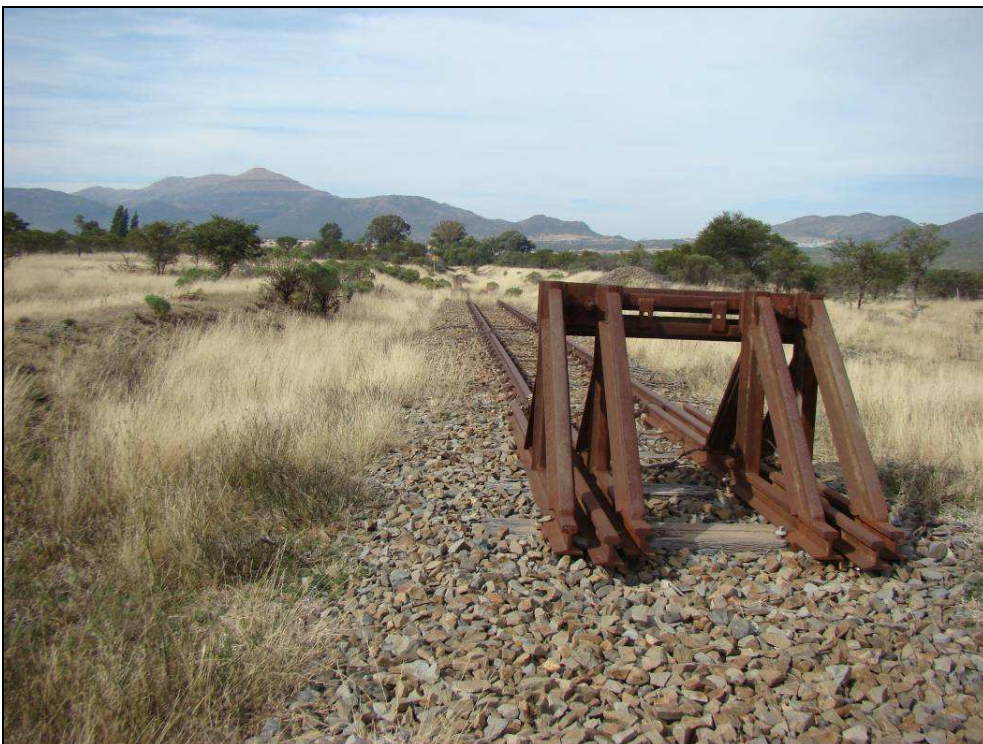
Fig.11 Point D. Railway line stop at the junction or office site.
