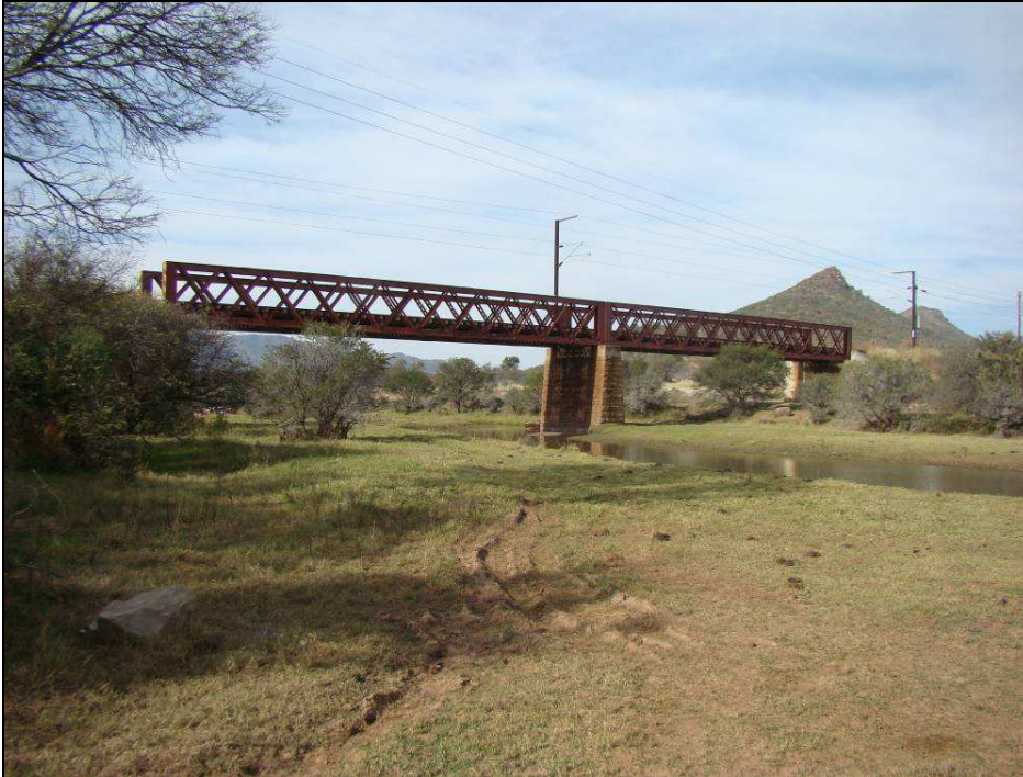
Fig.22 Bridge across the Lesseyton River near Bowkwer's Park siding.
