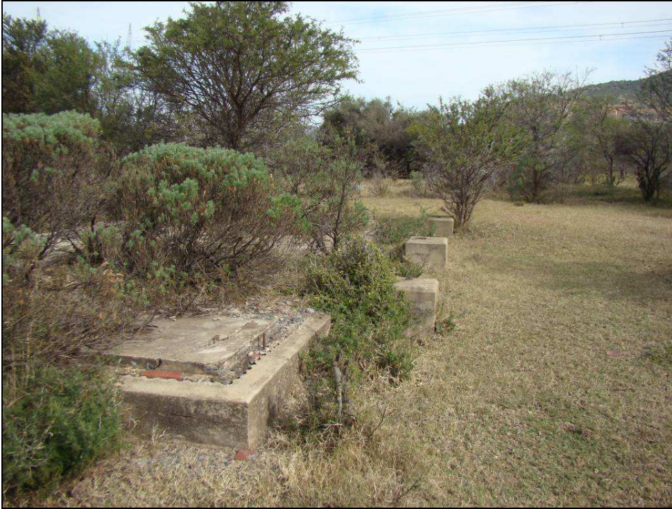
Fig.14 Point R. Remains of steel structure over bore hole.
