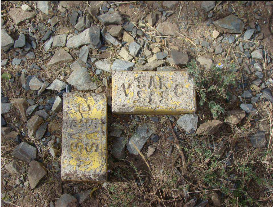
Fig.18 Remains of South African Railways underground cable layout.
