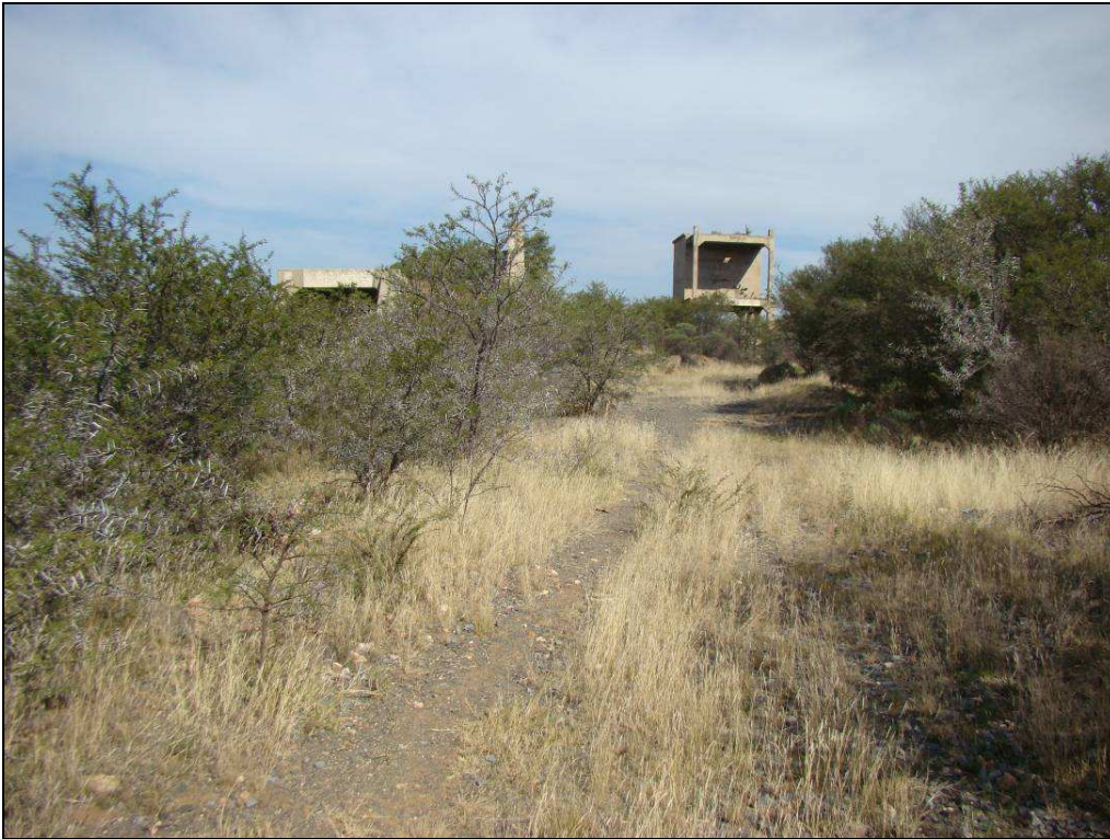
Fig.6 Point C near the loading bay at Bowker's Park quarry.
