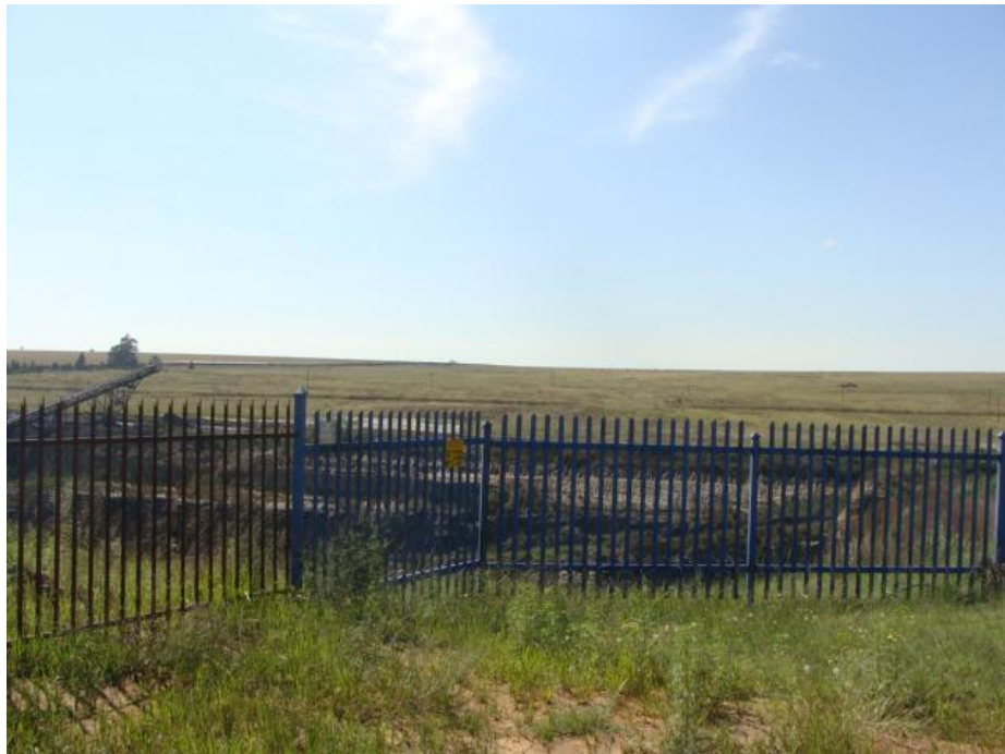
Figure 7 General view of the surveyed area including old mining infrastructure.
