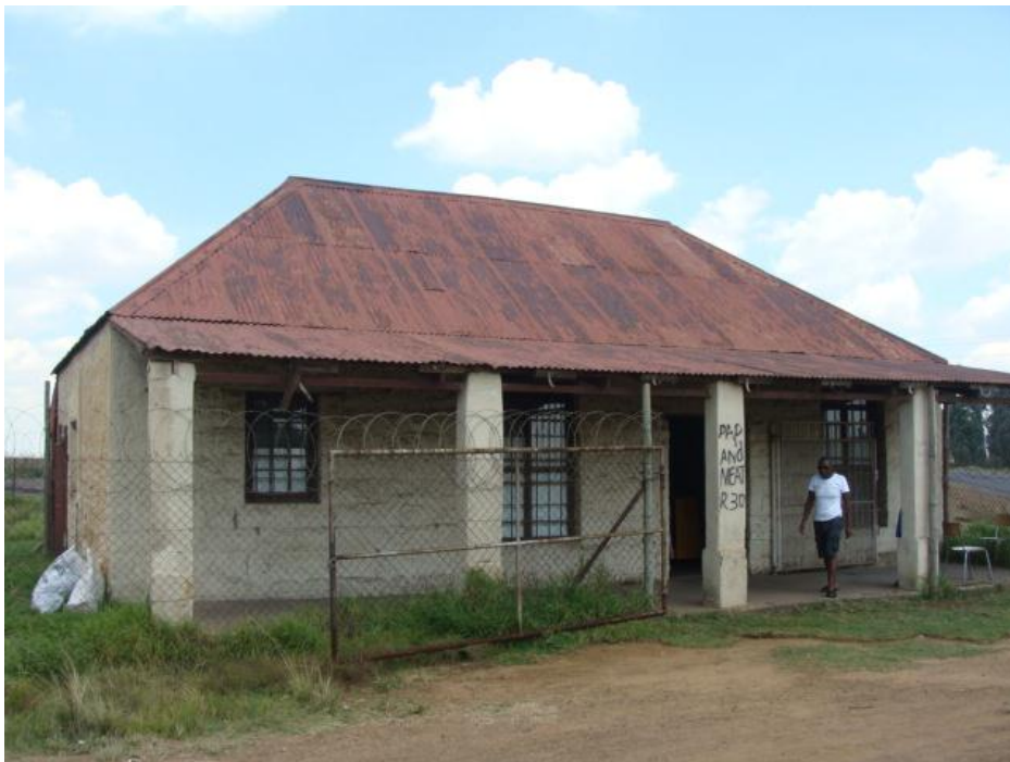
Figure 14 Building that apparently used to be an old post office at site no. 2.
