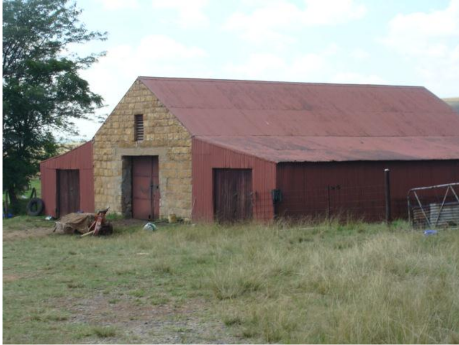
Figure 15 The wagon house at site no. 2.
