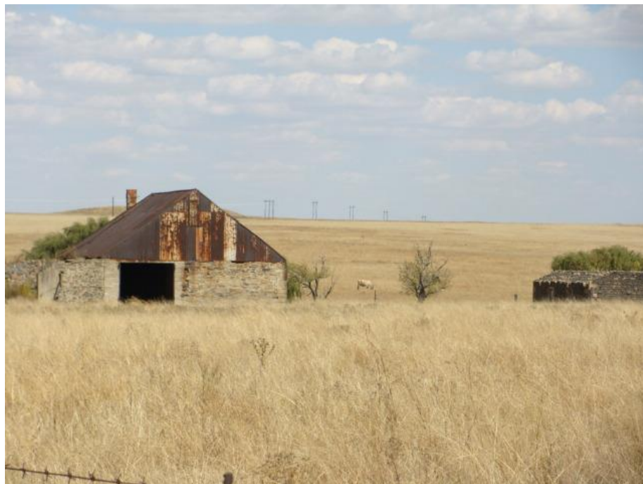
Figure 11 One of the outbuildings, most likely a wagon shed, at site no. 2.
