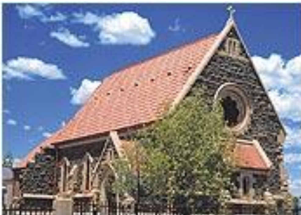
Figure 27 The former Anglican Church in Noupoort which now hosts a military museum.
