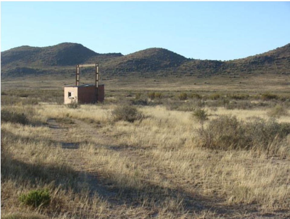
Figure 25 The Northern section ends at another borehole.
