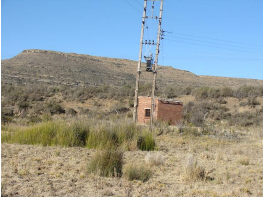
Figure 14 View of the area close to the end of the south-eastern section.
