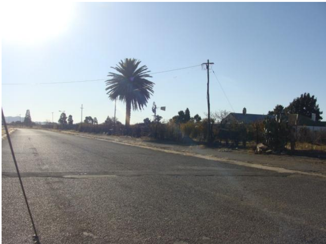
Figure 21 Section of road within the town, where the Northern section starts.
