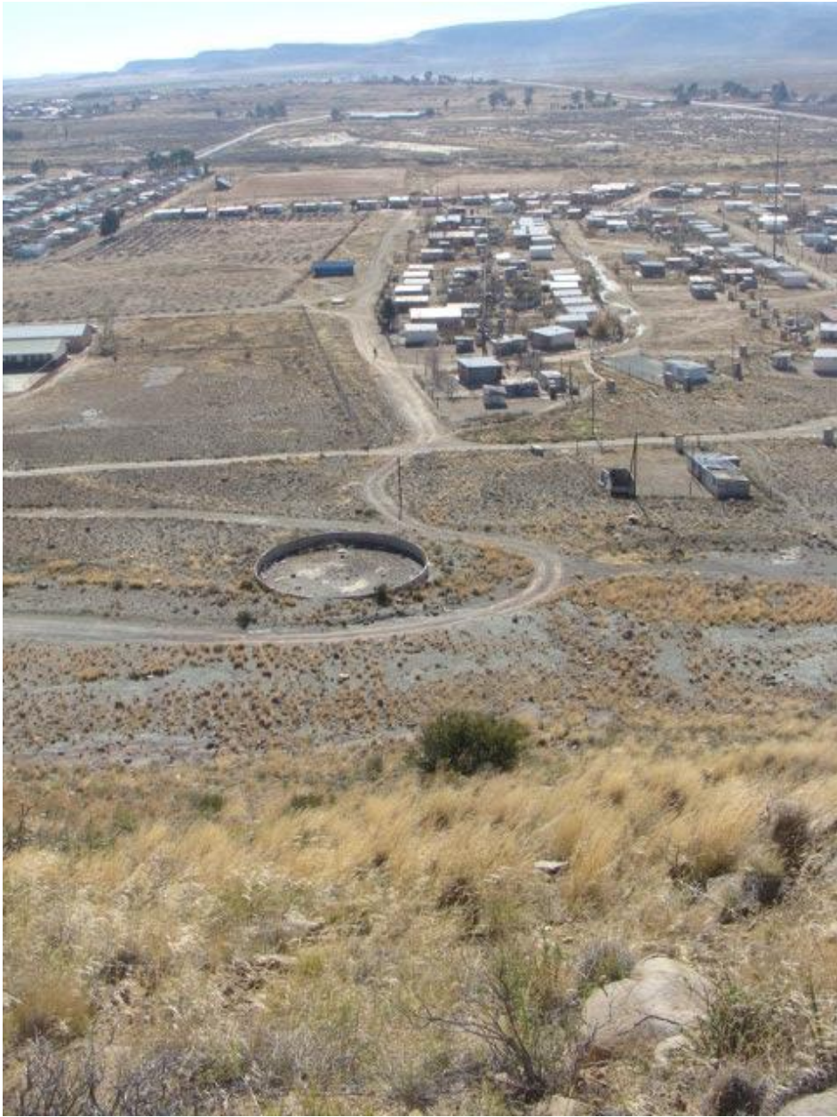
Figure 7 View of the town in the direction where the Central route will run.
