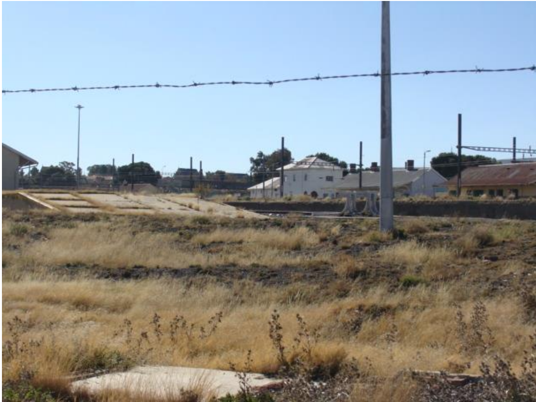
Figure 10 Disturbed area along the railway track where the central route will end.
