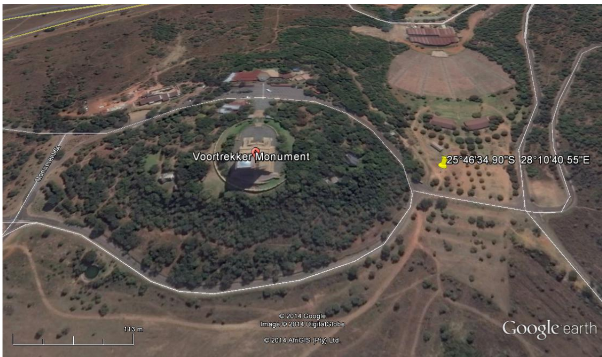
Figure 10 Specific location of the proposed development on the opposite side of the ring road around the Voortrekker Monument.
