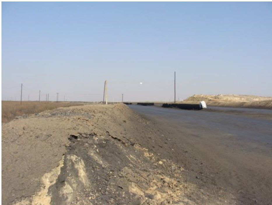
Figure 6: Mine road along which a short section of the proposed North Road will run.
