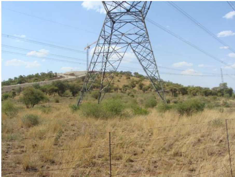
Figure 14: General view of the area where the bulk water route alternative 2 starts.
