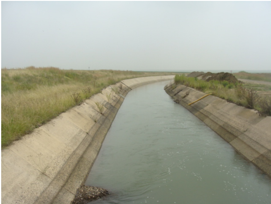
Figure 18: Irrigation canal in the surveyed area.
