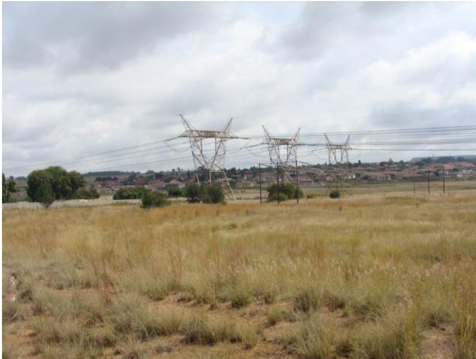
FIGURE 10: GENERAL VIEW OF AREA WHERE THE PROPOSED POERLINE ROUTE STARTS, CLOSE TO THE MRD.
