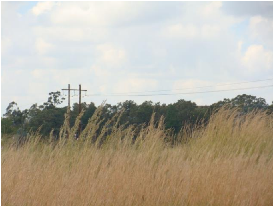
FIGURE 12: GENERAL VIEW OF VEGETATION ALONG THE POWER LINES ADJACENT TO THE N12.
