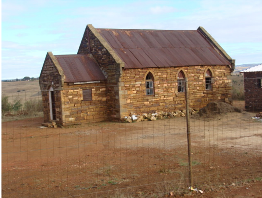
FIGURE 23: ANOTHER CHURCH BUILDING ALONG THE ROUTE IN KWATHANDEKA.
