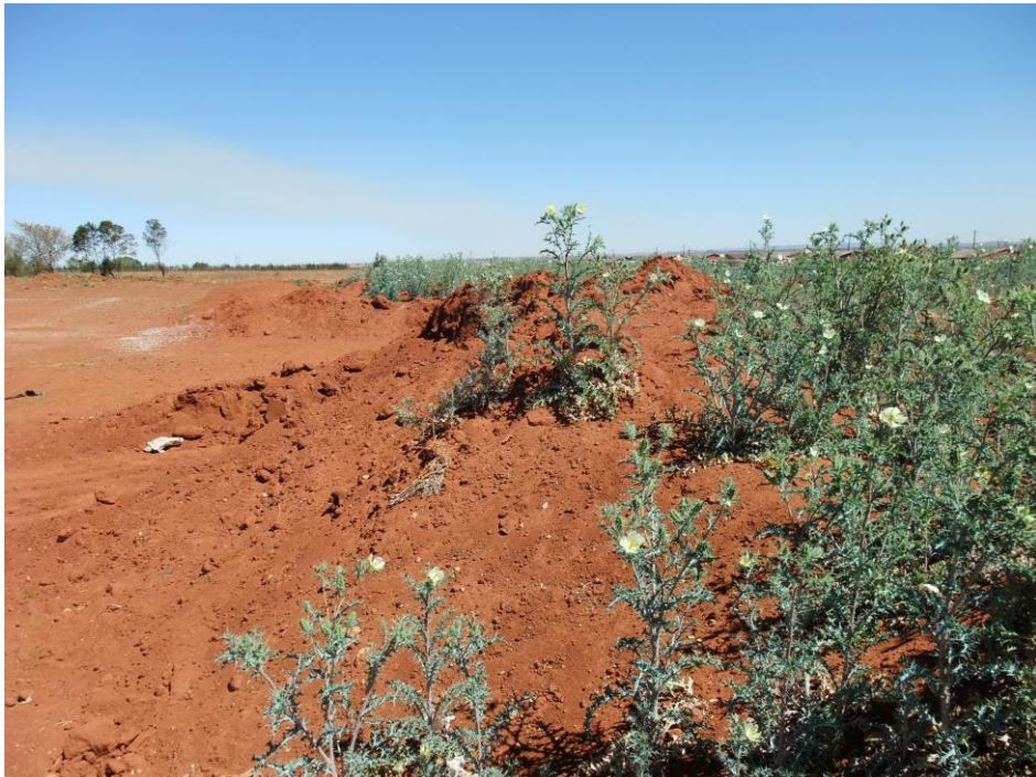
FIGURE 10: AREA SHOWING EARTH WORKS AND WEEDS.
