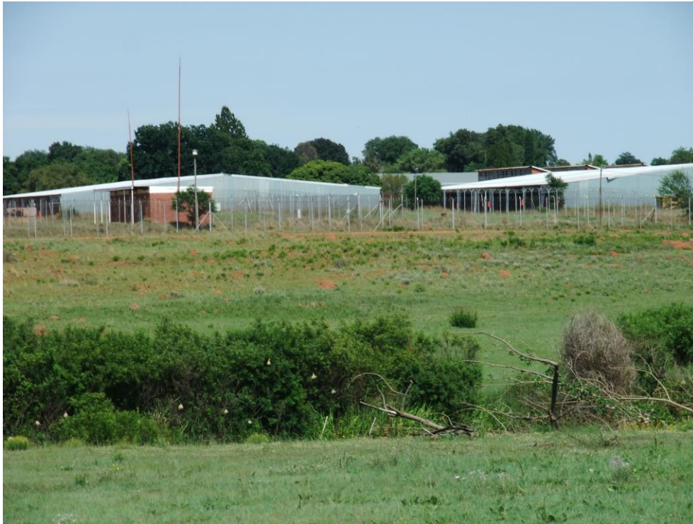
FIGURE 10: GENERAL VIEW OF THE SECTION BETWEEN THE RIVER AND THE SA NATIONAL DEFENCE FORCE PROPERTY.
