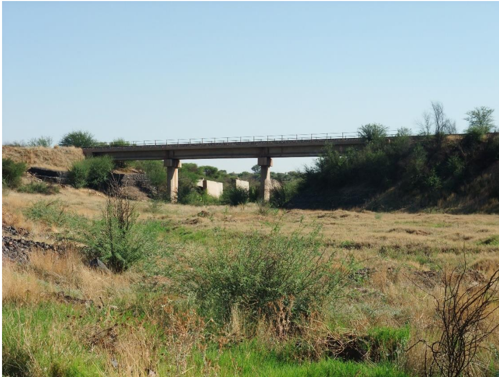
Figure 8: View of the area where the new bridge will be erected, next to the current one. Also note the pillars of a previous bridge.
