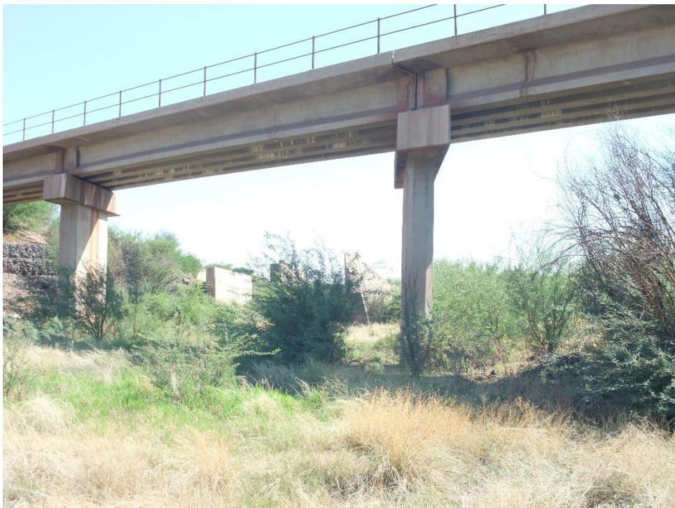
Figure 9: Closer view of the bridge.
