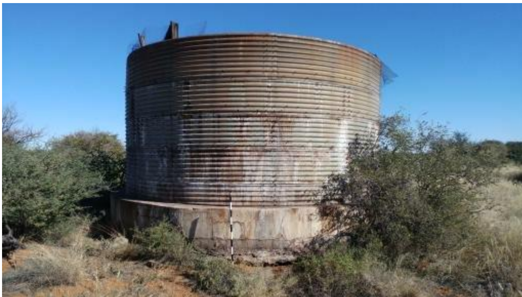
Figure 7: View of dam at the preferred location.
