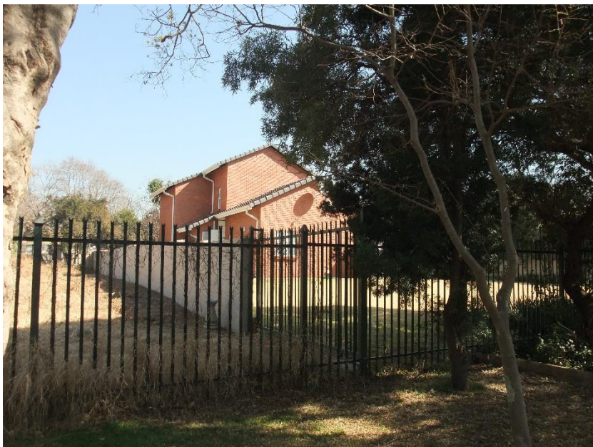
Figure 16: View towards the west. This is an open erf and one with a house which is younger than 60 years of age.
