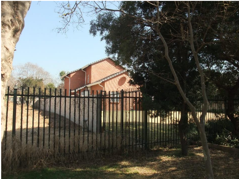
Figure 16: View towards the west. This is an open erf and one with a house which is younger than 60 years of age.
