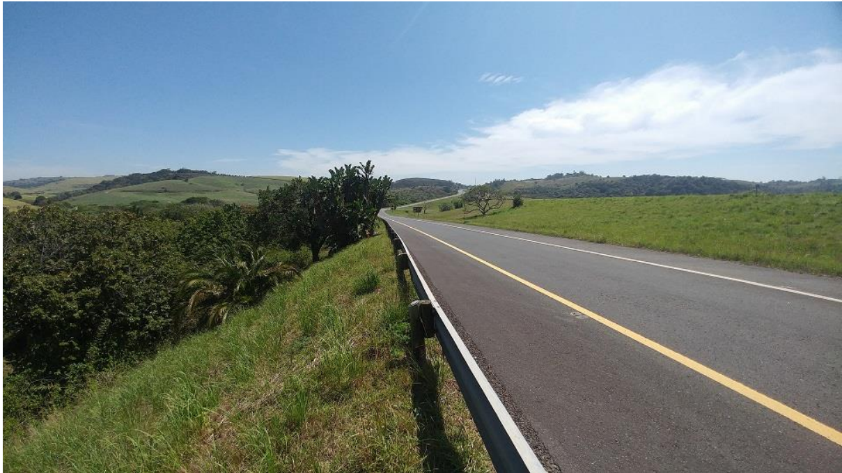
FIGURE 9: N2 HIGHWAY OFFRAMP EAST OF THE SURVEYED AREA.
