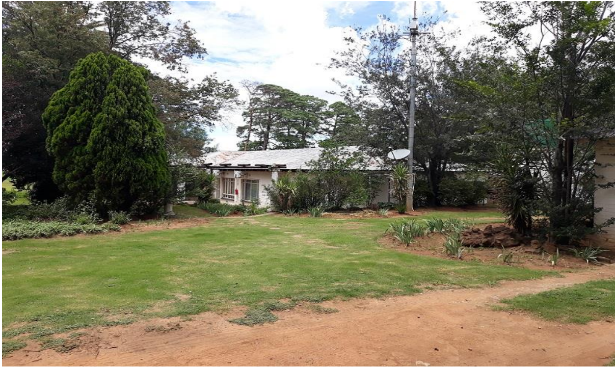
FIGURE 21: OLD FARMHOUSE INDICATING MANY CHANGES DONE DURING THE RECENT PAST.
