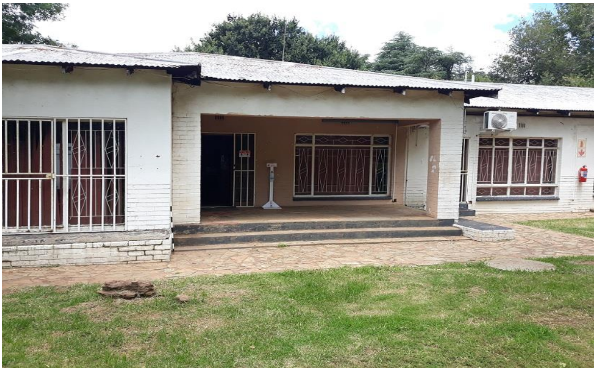
FIGURE 9: FARMHOUSE USED AS OFFICE.
