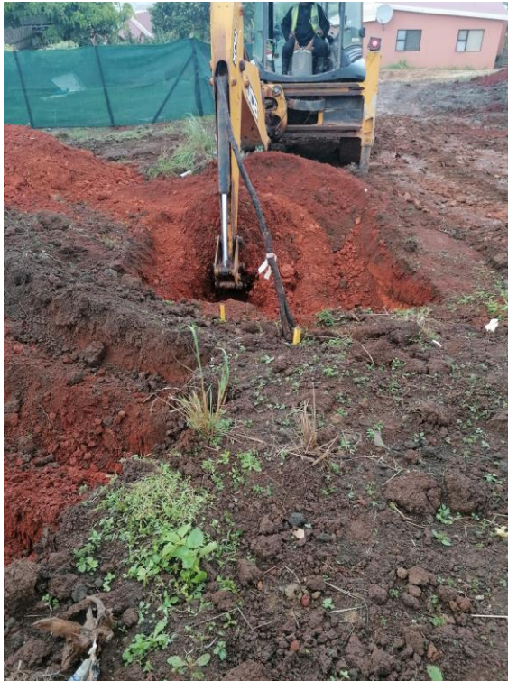
Figure 5: The excavator that was used.
