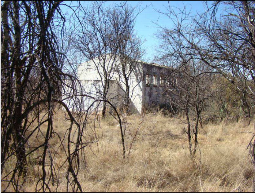
Fig.23 The old ablution block near the Boskop Dam, Potchefstroom.
