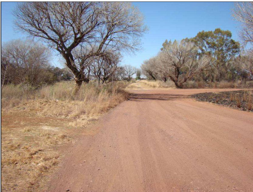
Fig.14 Point H at Boskop Dam, Potchefstroom.
