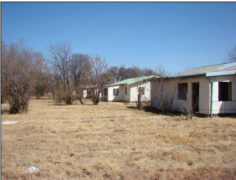
Fig.4 Abandoned pre-fabricated houses at Point B at Boskop Dam, Potchefstroom.
