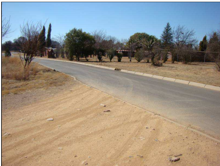
Fig.2 Point A facing existing office facilities at Boskop Dam.
