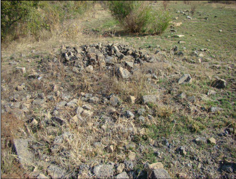
Fig.10 House rubble at the Bothaville ethanol plant site.
