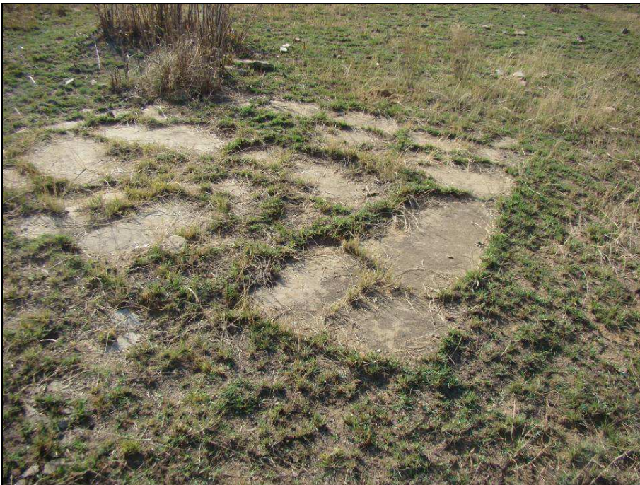
Fig.13 Concrete floor at the Bothaville ethanol plant site.
