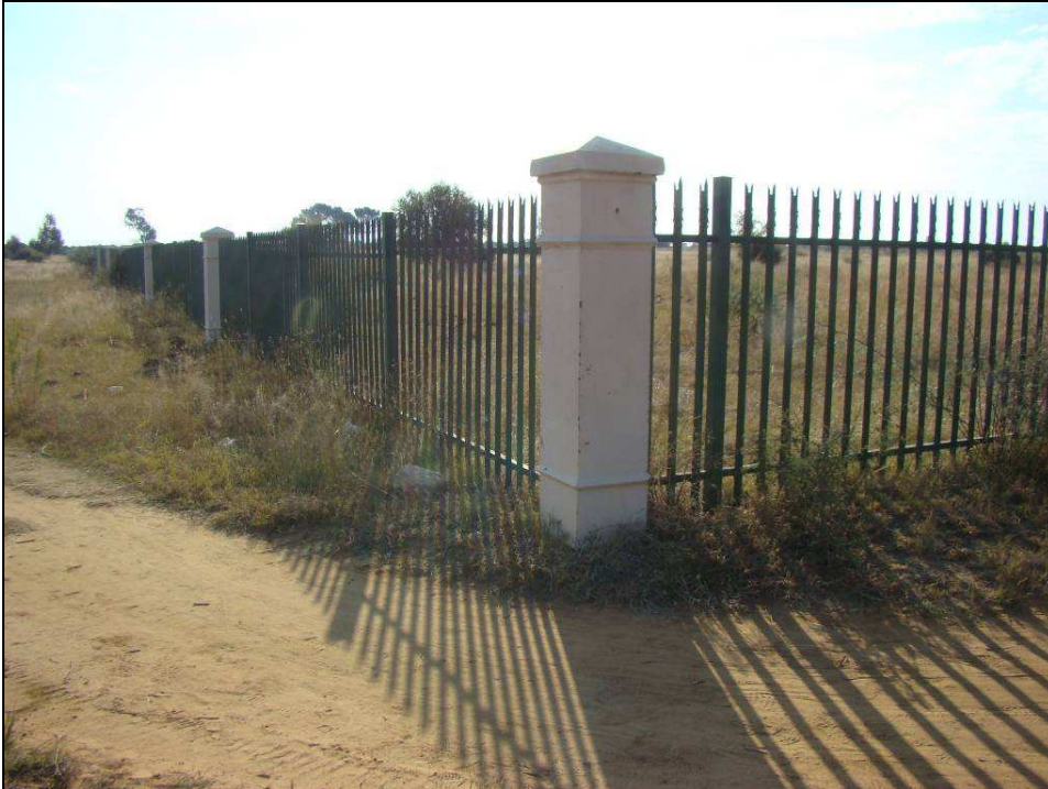
Fig.8 Point C at the Bothaville ethanol plant site.
