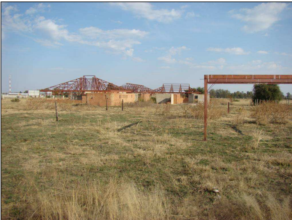
Fig.17 Ransacked structures at the Bothaville ethanol plant site.
