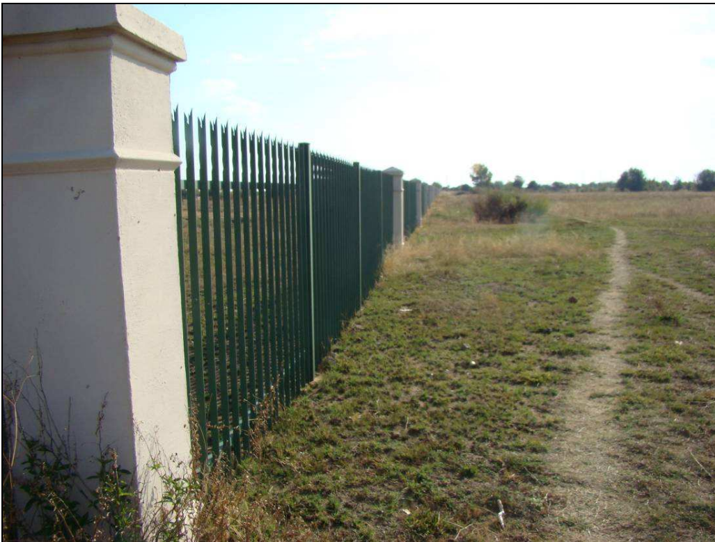
Fig.7 Point F at the Bothaville ethanol plant site, facing Point E along the devil's fork palisade.
