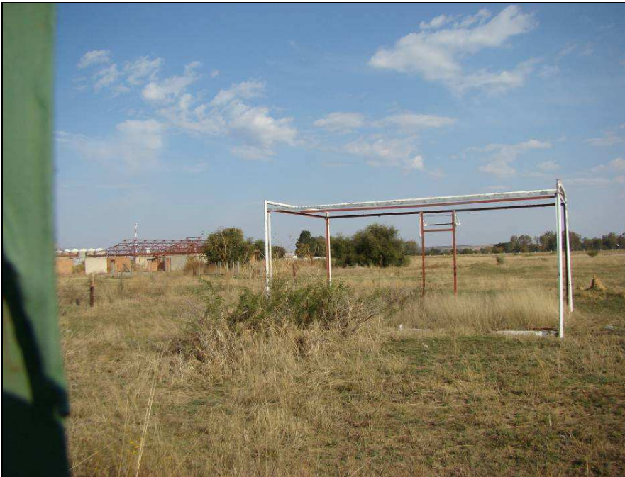
Fig.15 Stripped structures at the Bothaville ethanol plant site.
