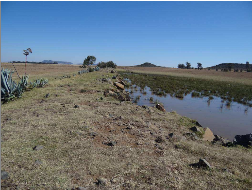
Fig.16 Dam wall at Point D at Brandkop farm.
