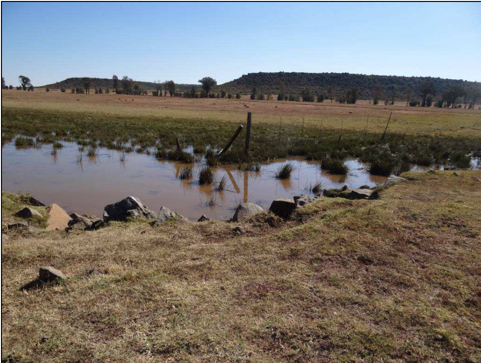
Fig.17 Dam wall at Point D at Brandkop farm.
