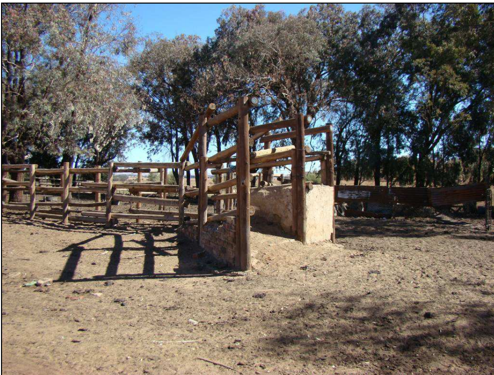
Fig.22 Stock loading bay at the site.
