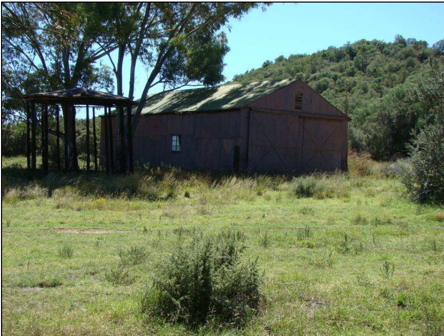
Fig.4 Corrugated iron shed.
