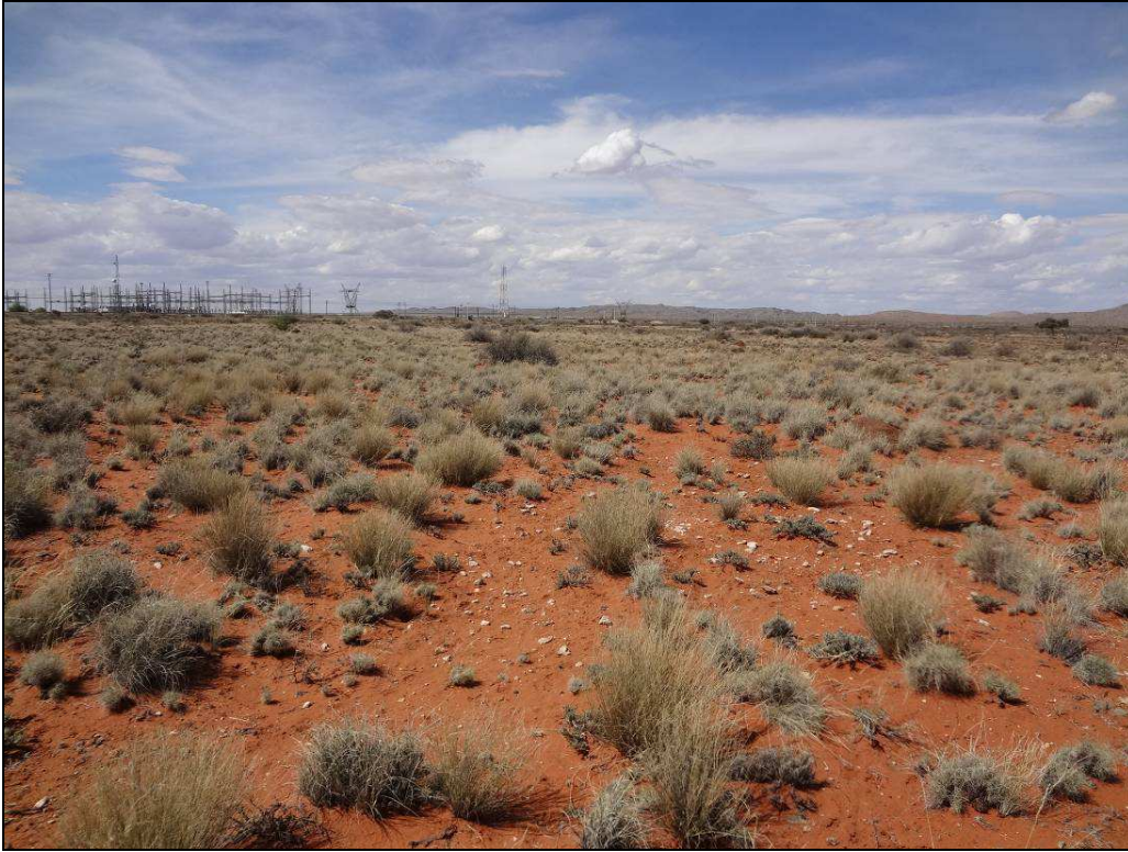
Fig.11 Pylon 360. Garona Sub-station at the back.
