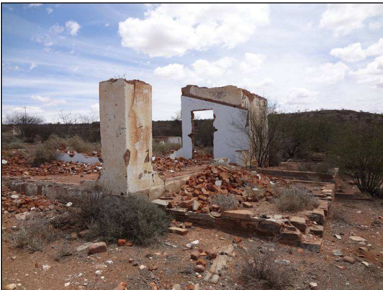
Fig.65 Abandoned farmhouse near Pylon 393 on the Orange River. Date of occupation is unknown.
