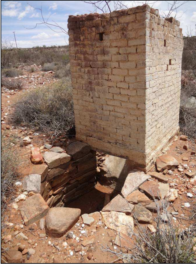
Fig.64 Inventive closet design at ruined farmyard near Pylon 393. Note sloping floor inside with external stone built septic tank.
