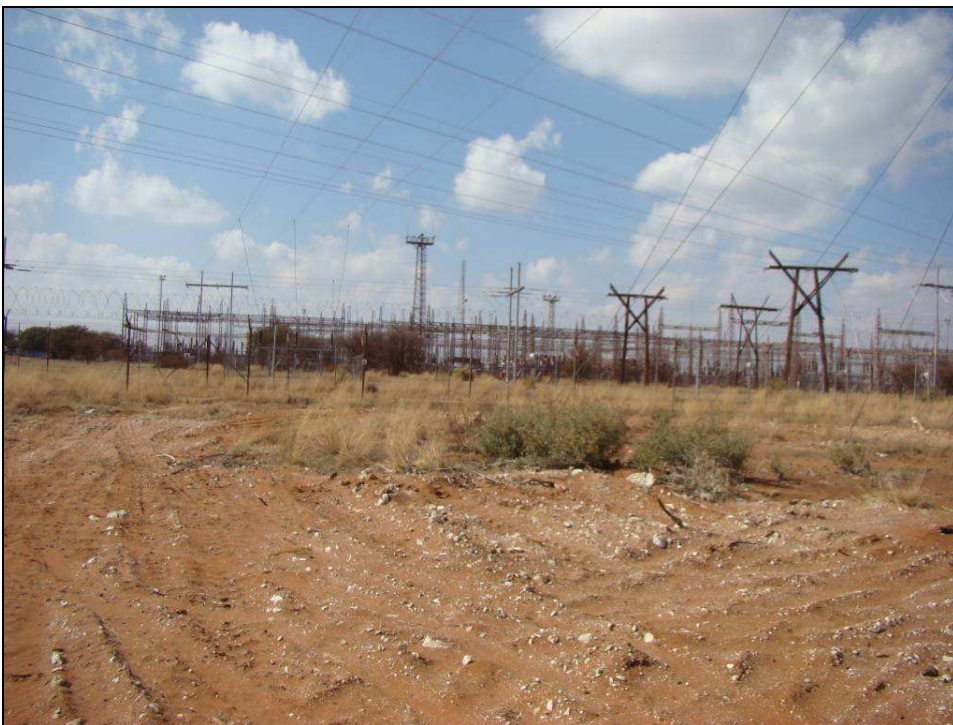
Fig.14 Pylon K6 at Ferrum outside Kathu.
