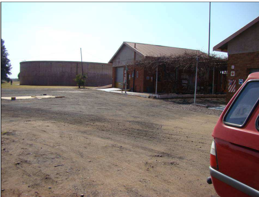
Fig.10 Water supply reservoir at Kathu.
