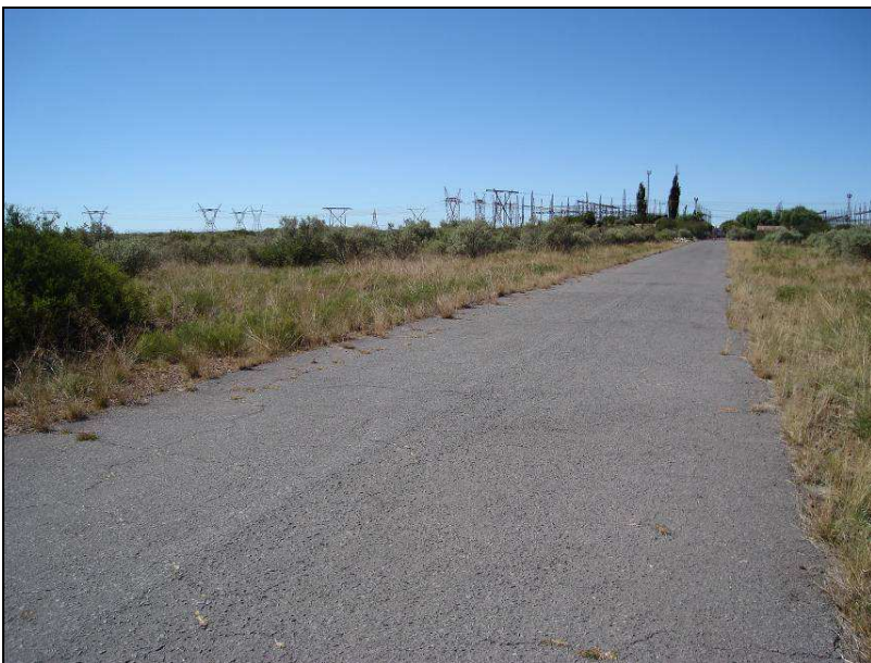
Fig.8 Point 12. Ferrum Sub-Station at Kathu.
