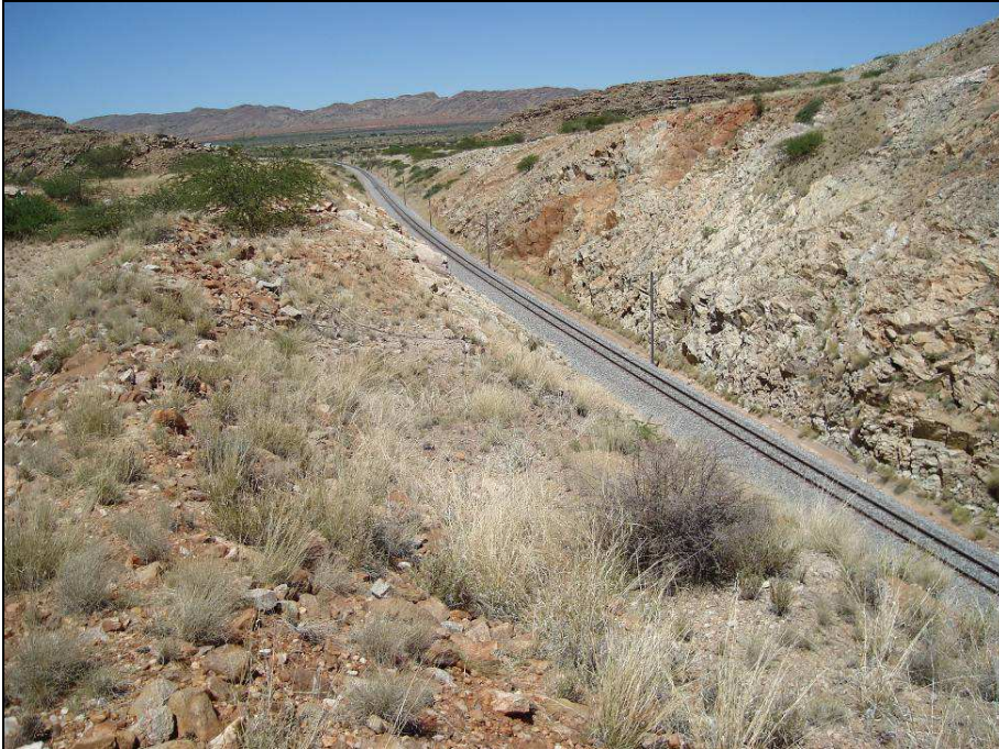
Fig.3 Point 2. The cutting for the railway line.
