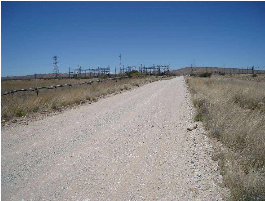
Fig.1 Garona Sub-Station near Groblershoop (Point 1 Map 10).
