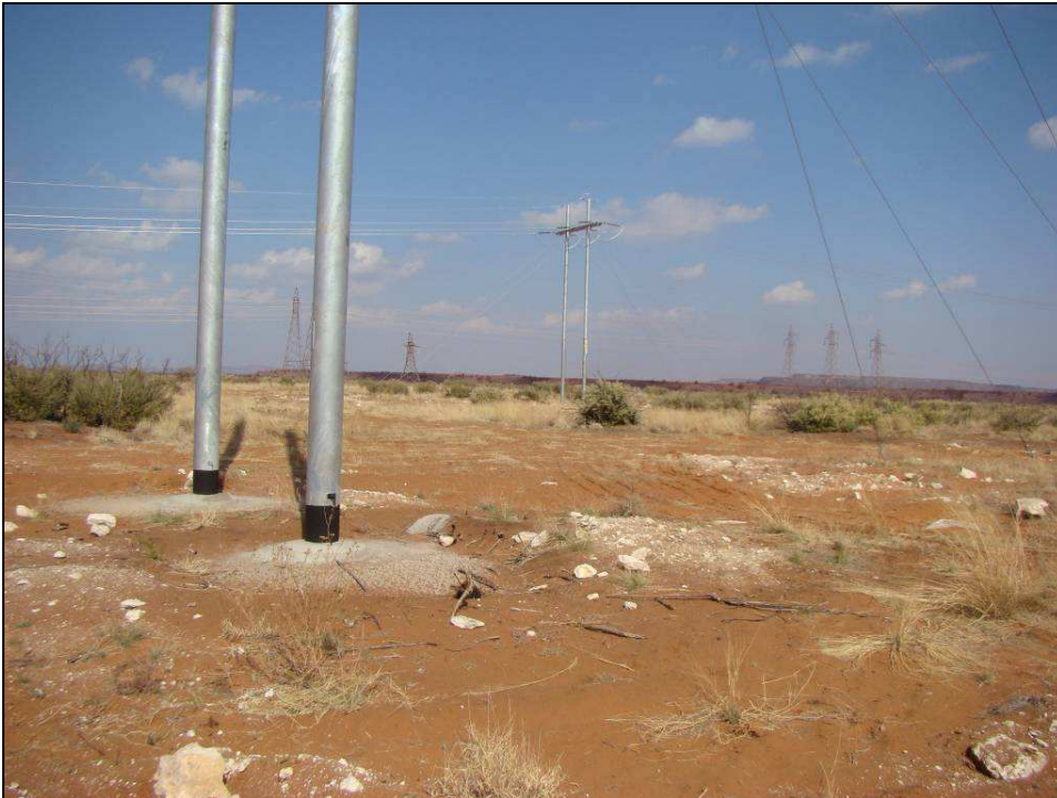
Fig.15 Pylon K6 at Ferrum outside Kathu.
