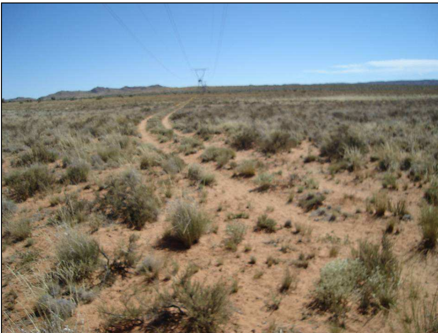
Fig.4 Point 4. Pylon 373 (735km).
