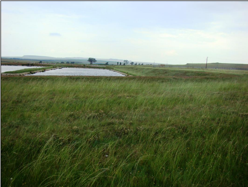
Fig.1 Sewer dams at Point A, Glen Lenie, Harrismith.
