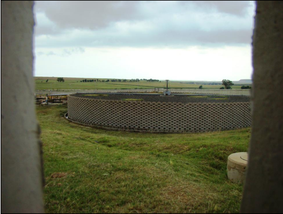
Fig.9 The sewer plant at Glen Lenie, Harrismith.
