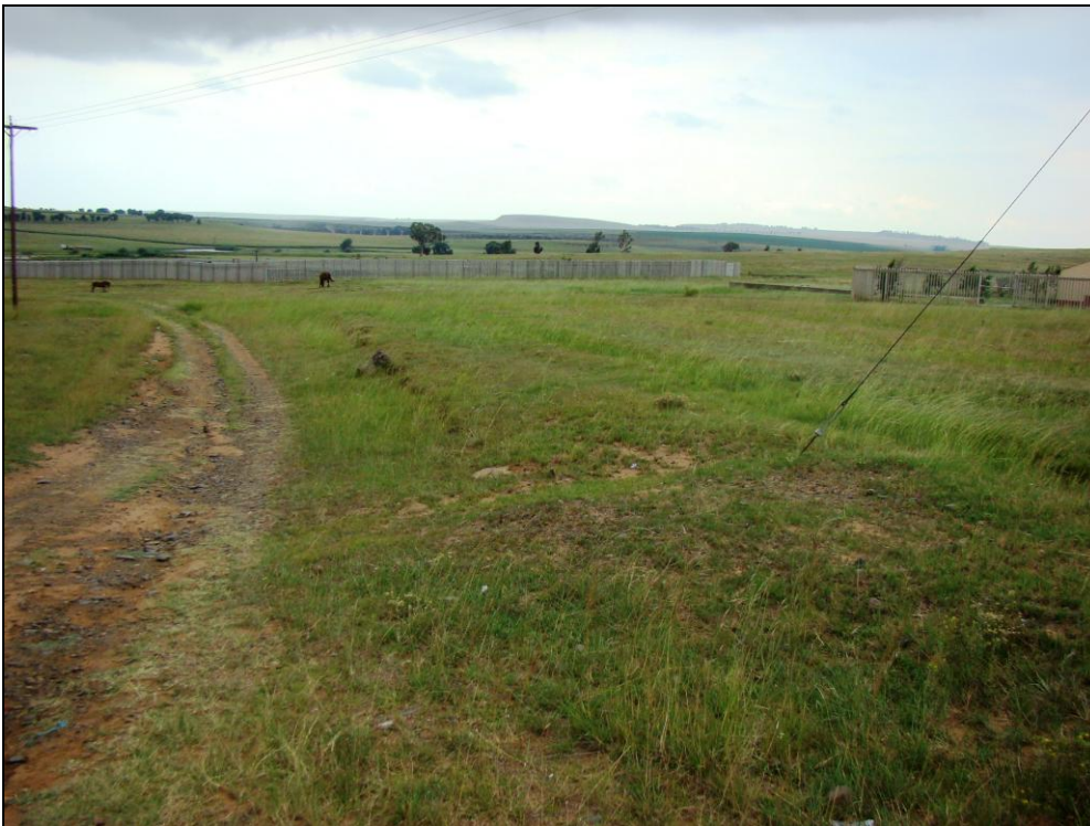
Fig.4 Point B facing the sewer plant at Glen Lenie, Harrismith.
