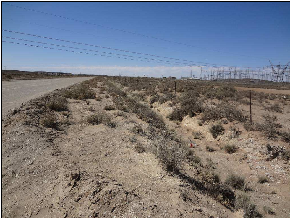
Fig.2 Helios Sub-station as seen from Point C.
