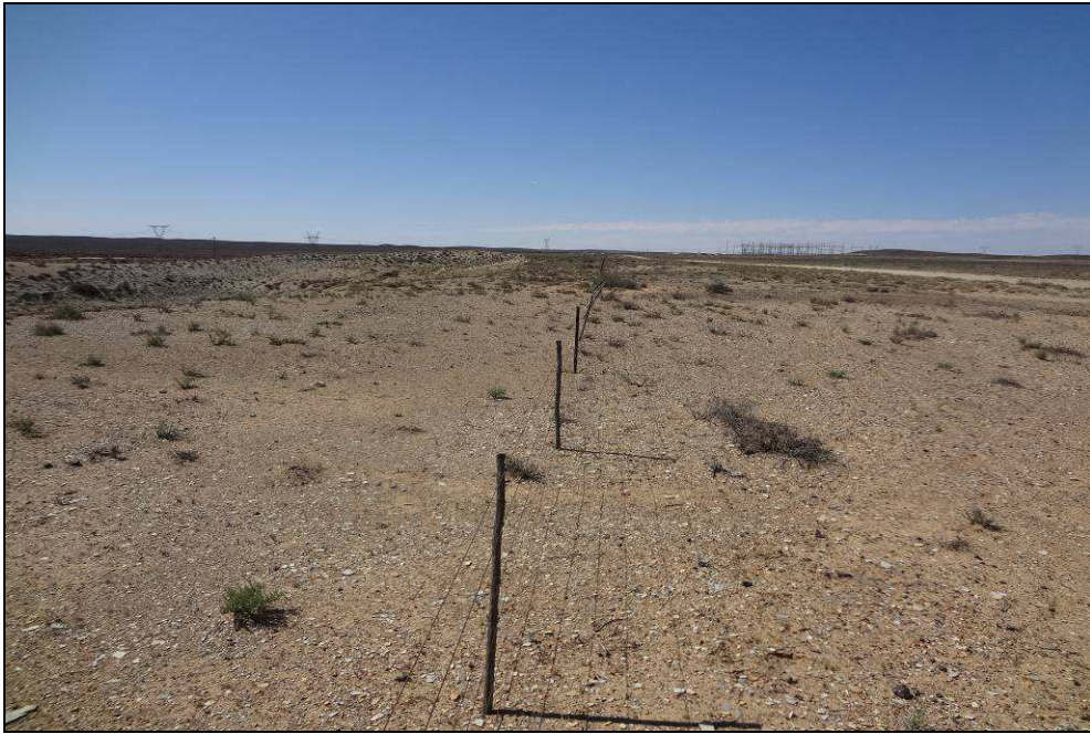
Fig.5 Point B near Eskom Helios Sub-station.
