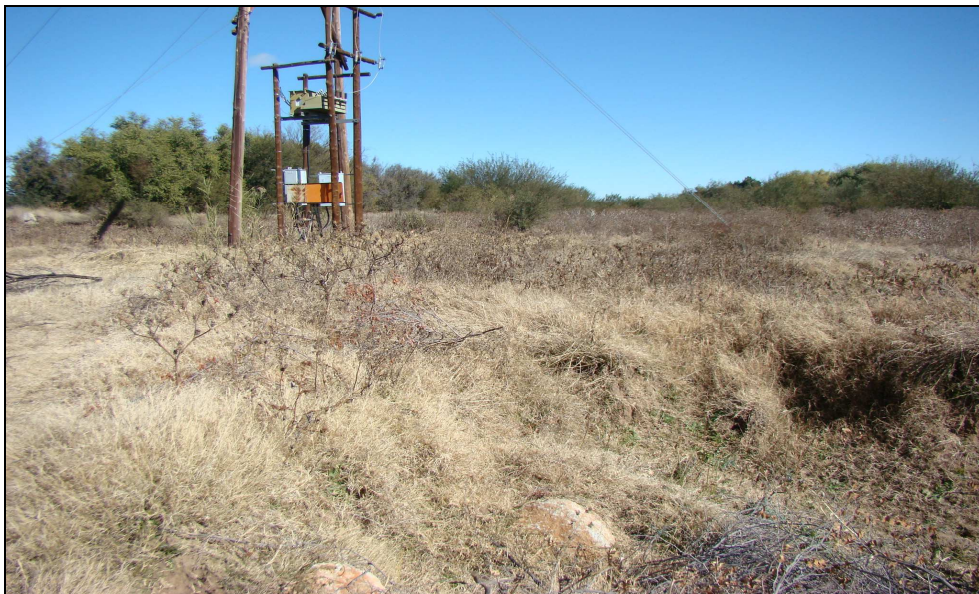
Fig.1 Point C at Melkstroom 563, Upington.
