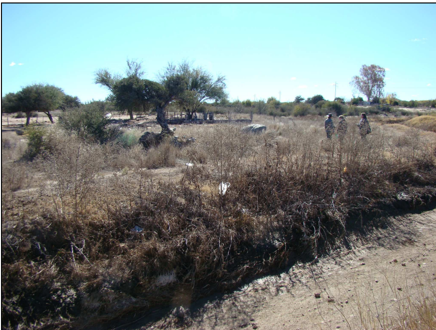
Fig.6 Flood water ditch at Point F, Melkstroom 563, Upington.
