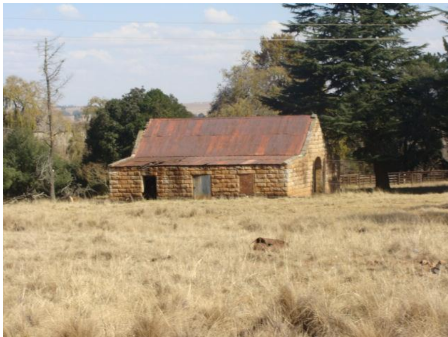
Figure 18 Wagon house (site 12) on the farm Meppel.
