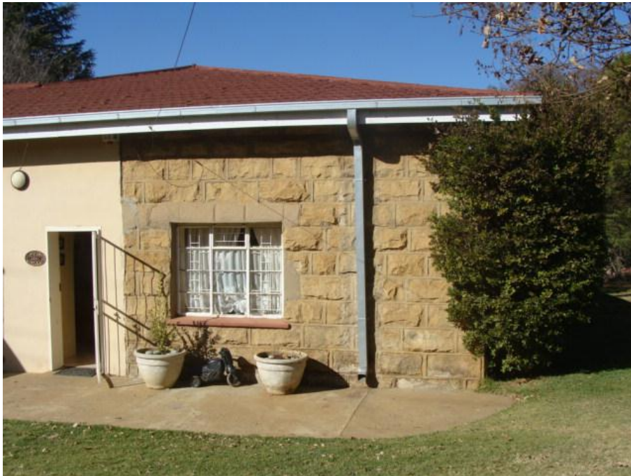
Figure 7 View of the farm house on Joubertsvei showing later additions.
