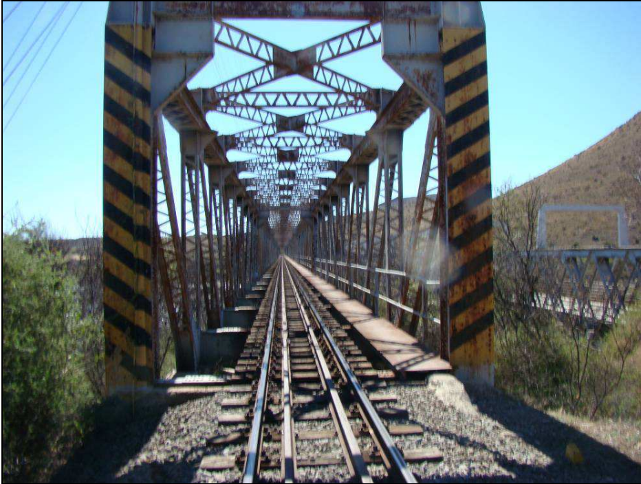
Fig.9 Railway bridge across the Orange River near the Norvalspont pump station.
