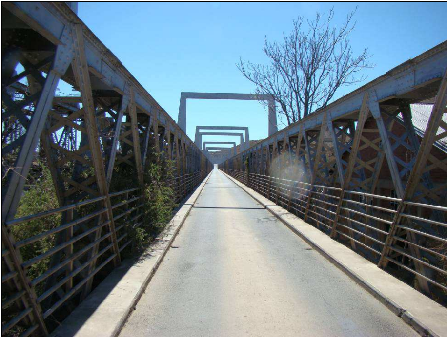
Fig.5 Road bridge across the Orange River near the Norvalspont pump station.
