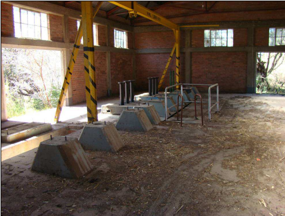
Fig.3 Interior of the old pump station building at the Orange River.
