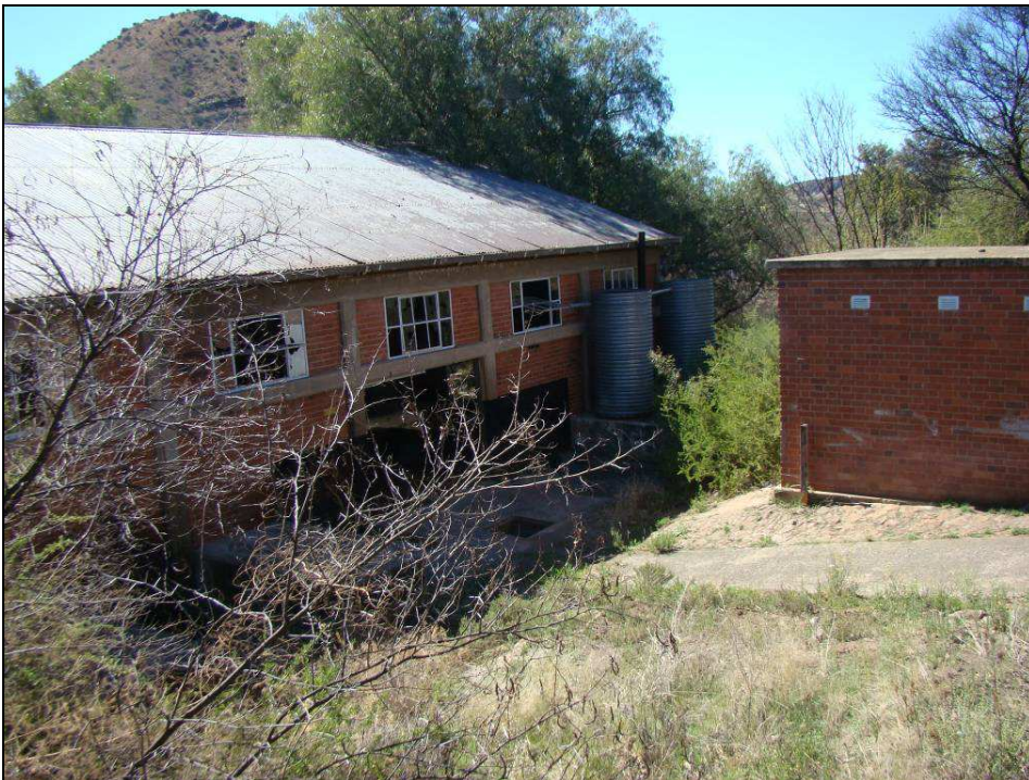
Fig.2 Old pump station building at the Orange River.
