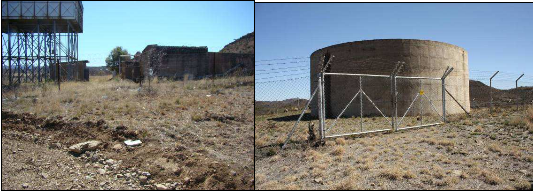
Fig.1 Reservoir at the water treatment works, Norvalspont.
