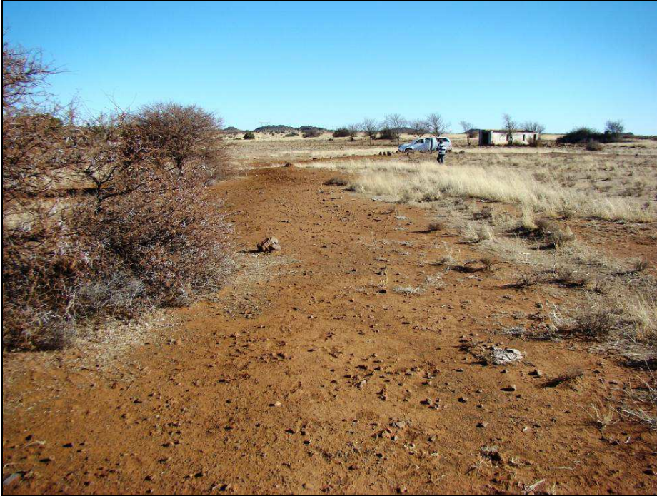
Fig.8 Point D at the dam wall Pretoriusdam 550, Petrusburg.
