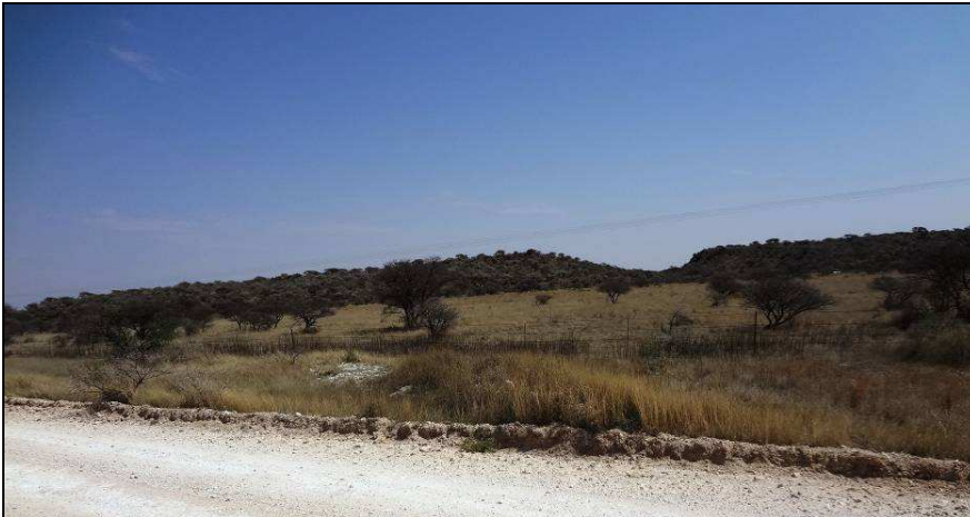
Fig.15 Point K along the Riverton – Boshof – Dealesville water pipeline.
