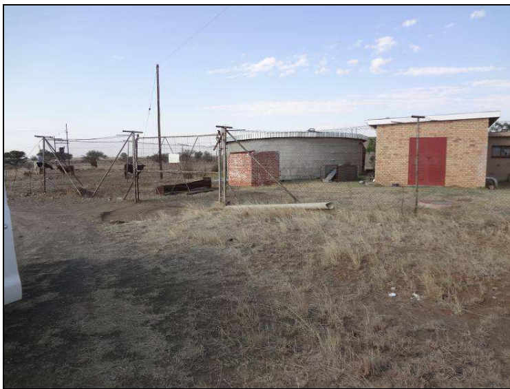
Fig.2 Water reservoir at Dealesville (Point DV).
