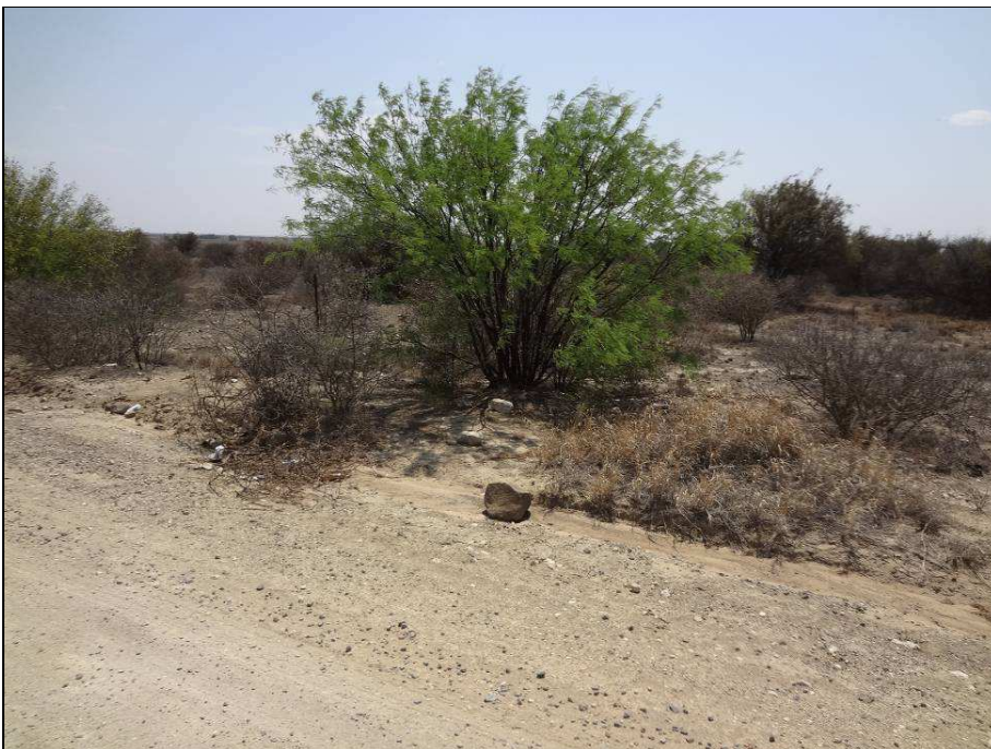
Fig.33 Point T (N12) along the Riverton – Boshof – Dealesville water pipeline.
