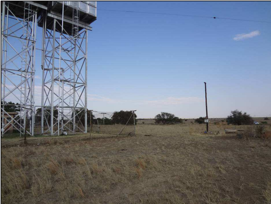
Fig.1 Water reservoir at Dealesville (Point DV).
