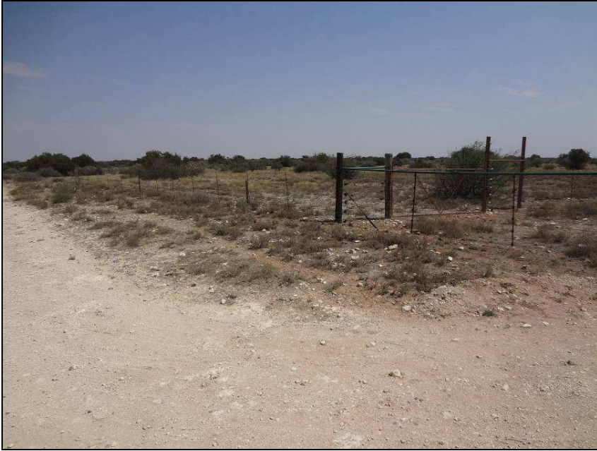
Fig.18 Point N along the Riverton – Boshof – Dealesville water pipeline.
