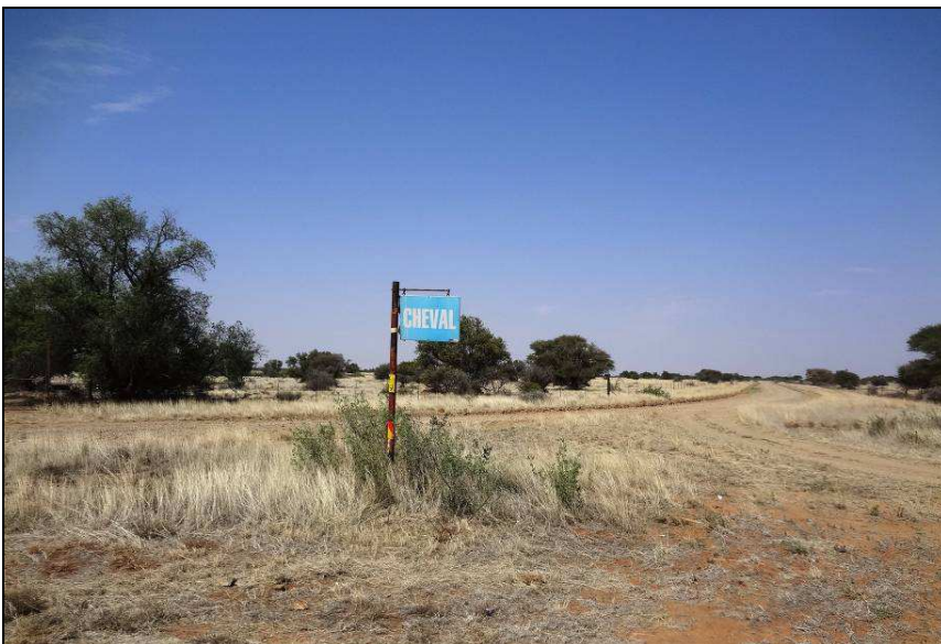
Fig.17 Point M (Cheval) Riverton – Boshof – Dealesville water pipeline (2825CA).
