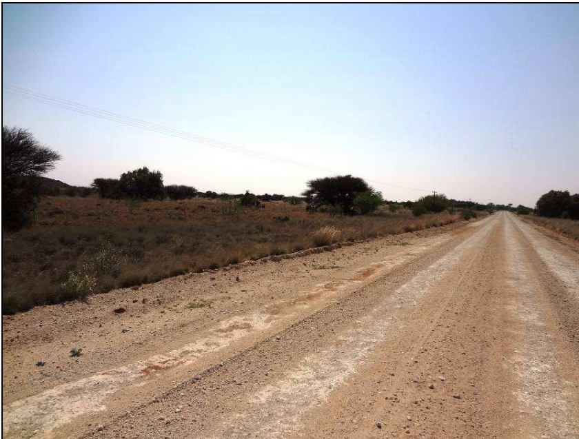
Fig.14 Point J along the Riverton – Boshof – Dealesville water pipeline.
