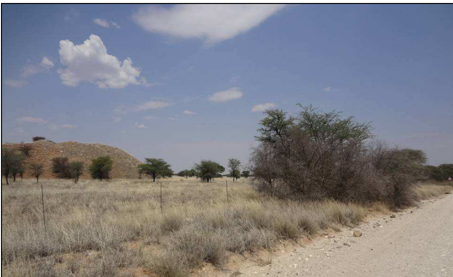
Fig.35 Point U along the Riverton – Boshof – Dealesville water pipeline.
