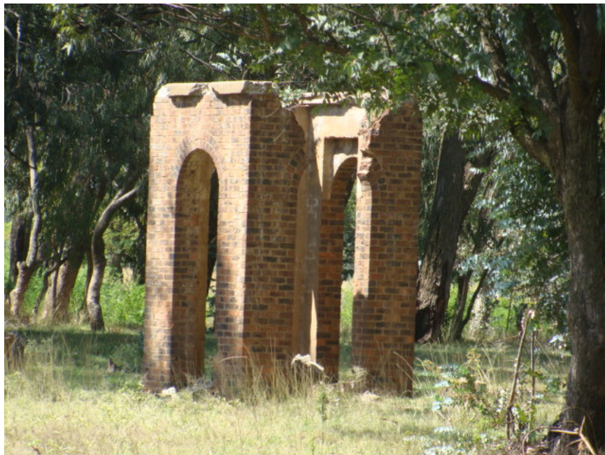
Figure 12 Face brick structure at site no. 6.
