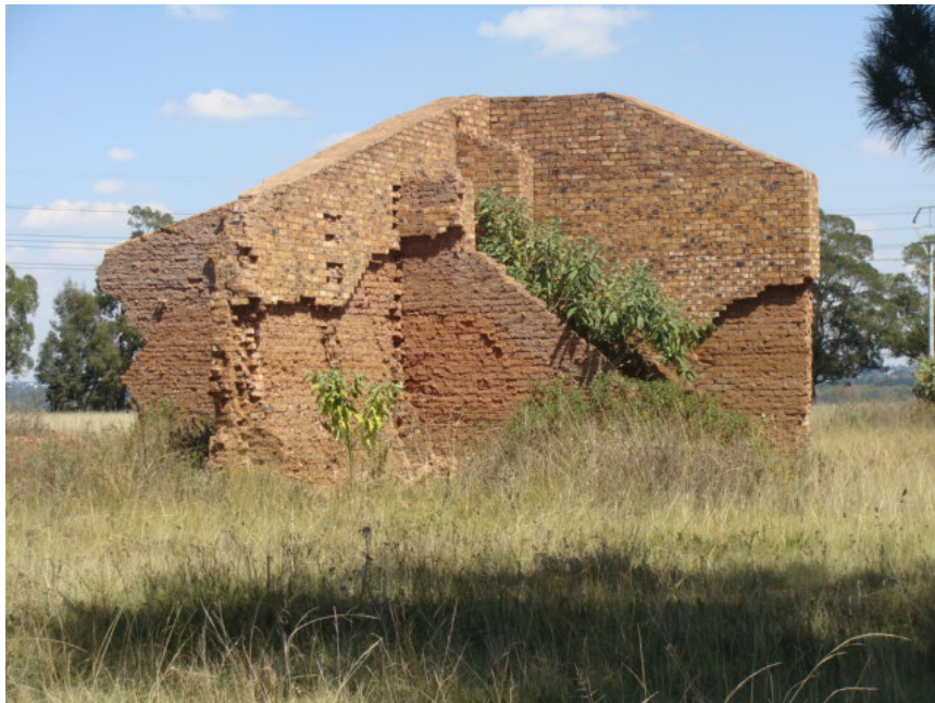
Figure 14 Industrial building at site no. 8.
