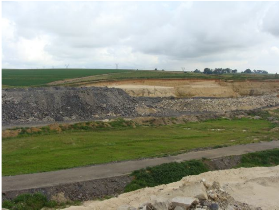
Figure 8 Another view of the surveyed area.
