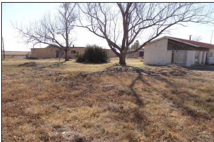
Fig.4 The existing buildings as seen from Point B at Palmiet 585, Vrede.
