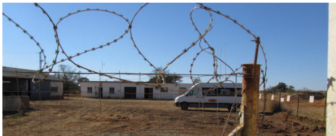
Figure 25. Workshops adjacent to the 1960's homestead farmyard. Some of these are new but others are part of the old farmyard's outbuildings.
