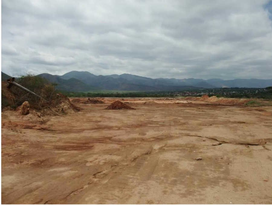
Figure 6: General view of TSF being reclaimed.
