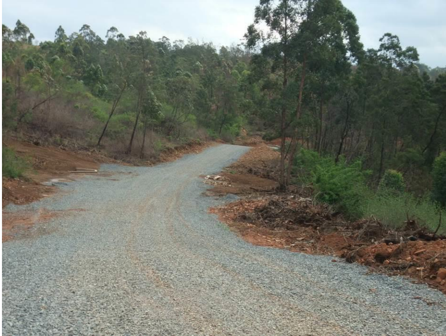
Figure 8: Section of road that will be upgraded.
