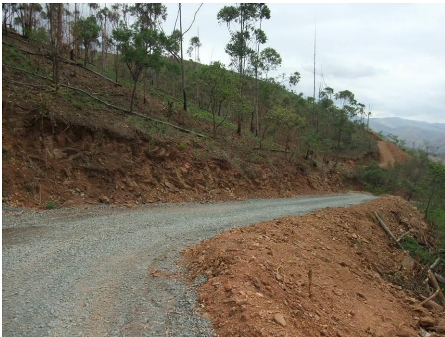
Figure 9: Another section of the road to be upgraded.
