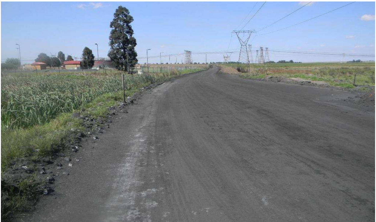
Plate 8: Photo 8: View of road servitude, Sewerage treatment plant and a network powerlines within the development area (Photograph © by Author 2017).
