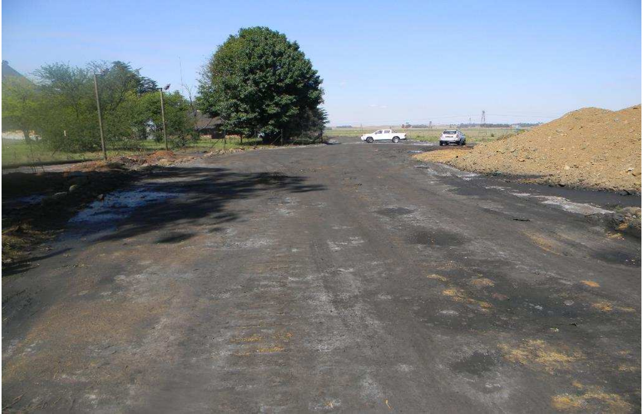
Plate 3: Photo 3: View of existing road earmarked for upgrading (Photograph © by Author 2017).
