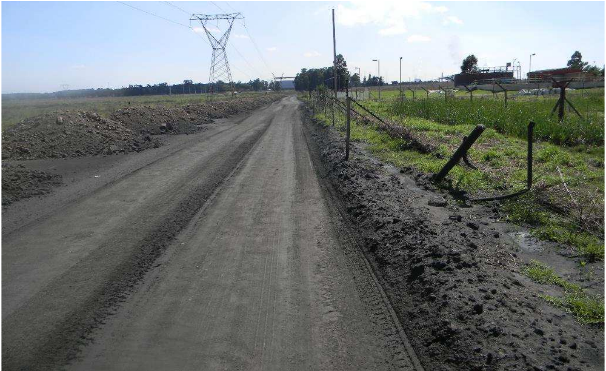
Plate 9: Photo 9: View of road servitude, and sewerage treatment plant on the right (Photograph © by Author 2017).
