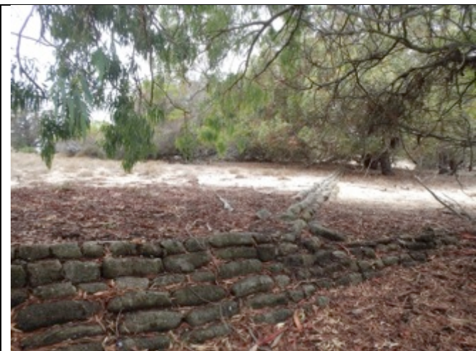
Figure 45: Second tier of sandbag terracing within the wattle plantation
