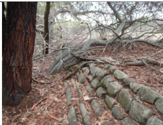
Figure 44: Terracing within the plantation showing some damage from tree growth.
