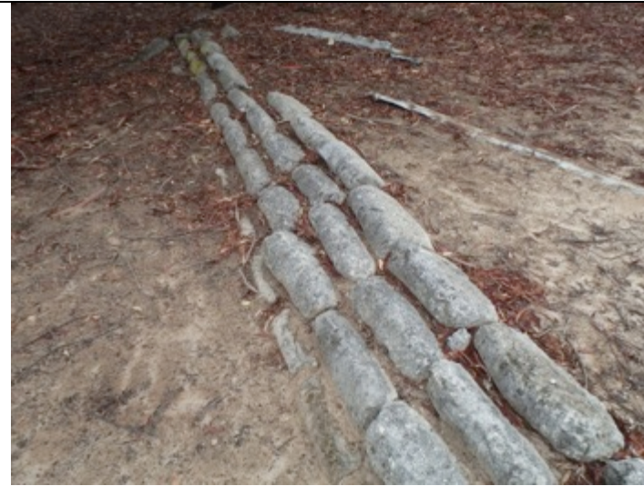
Figure 42: Terracing created with concrete sandbag formation within the wattle plantation
